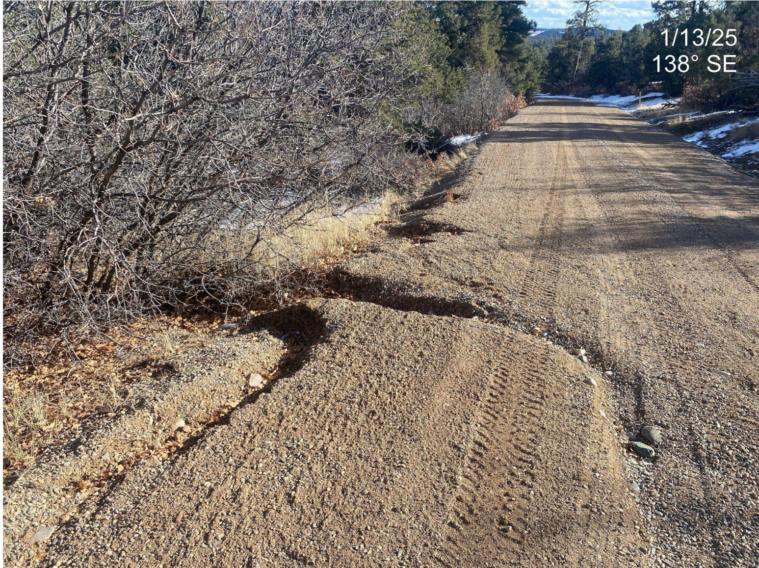
Photo 2. Erosion observed along access road.
