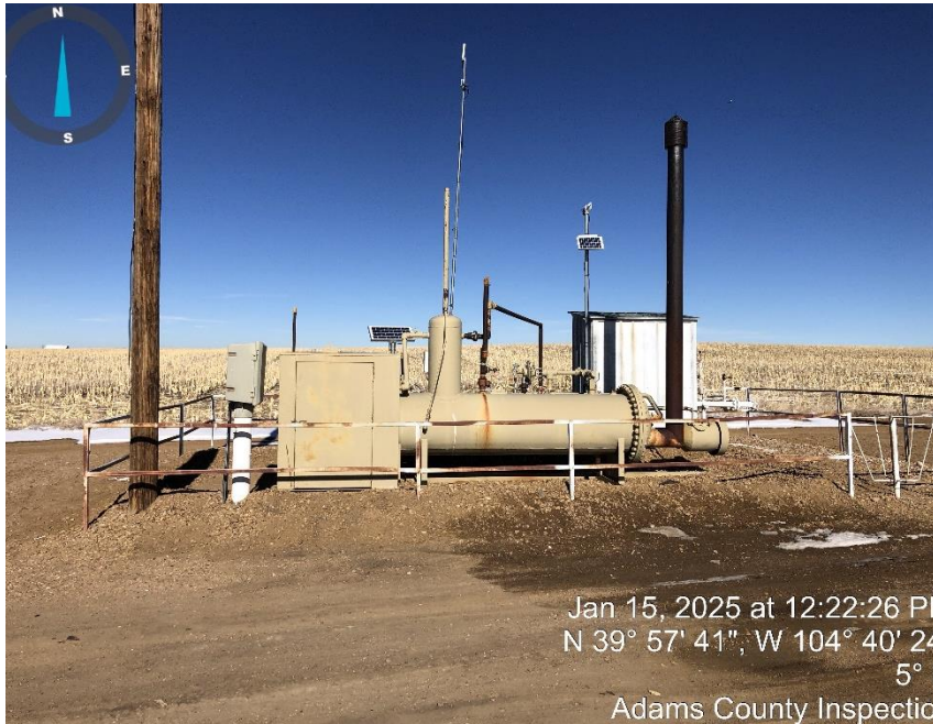
Photo #3 Meter & Separator.
