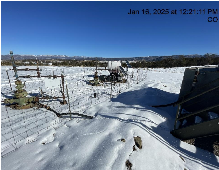
Photo # 9532 CIRCLE B LAND 14C-35-692 well bradenhead line connected to blowdown tank
