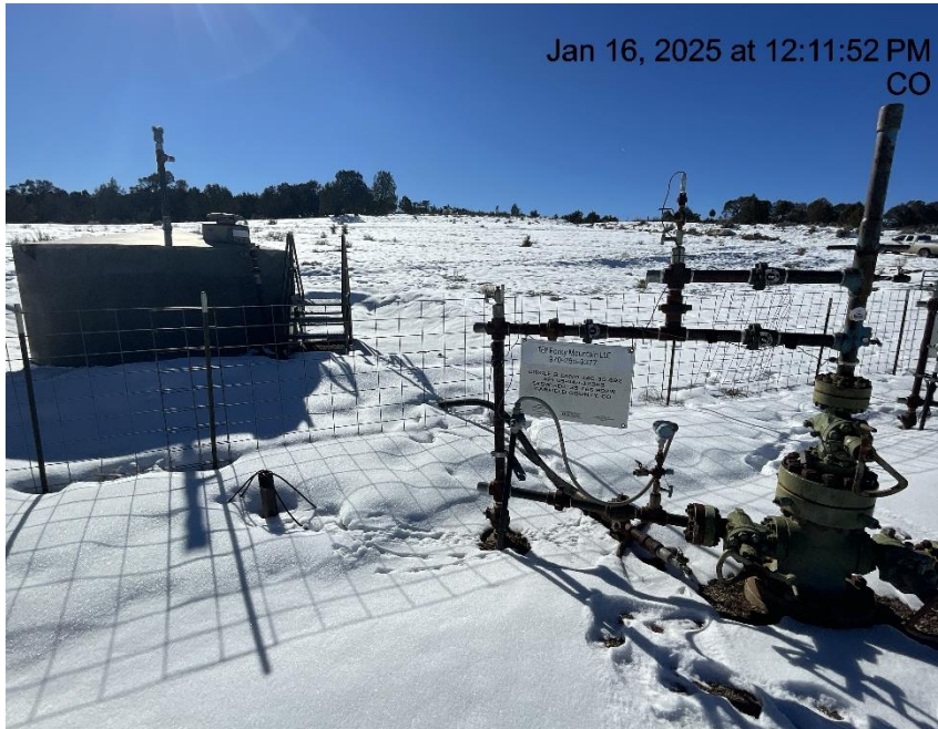
Photo # 9530 CIRCLE B LAND 14C-35-692 well bradenhead line connected to blowdown tank
