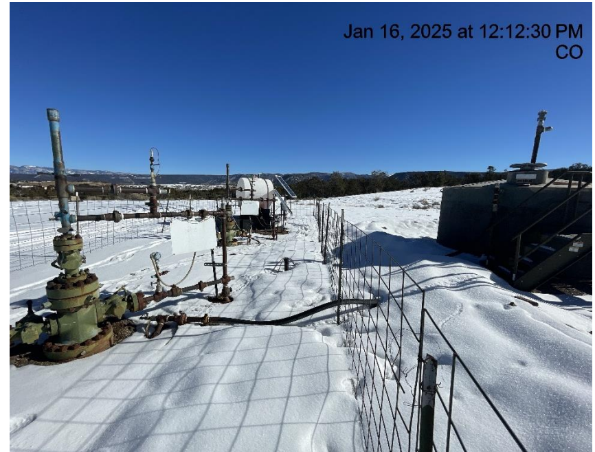
Photo # 9531 CIRCLE B LAND 14C-35-692 well bradenhead line connected to blowdown tank
