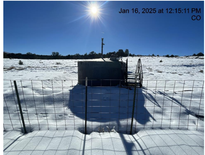
Photo # 9536 Secondary containment insufficient/does not comply with CECMC rules
