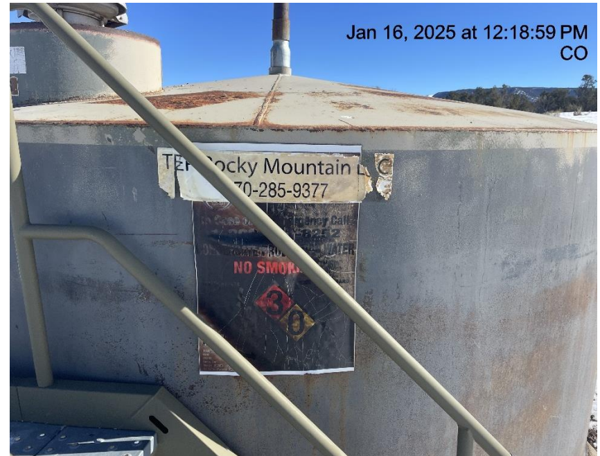
Photo # 9534 Blowdown tank label weathered & illegible /does not comply with CECMC rules. Additionally capacity on tank label is also incorrect
