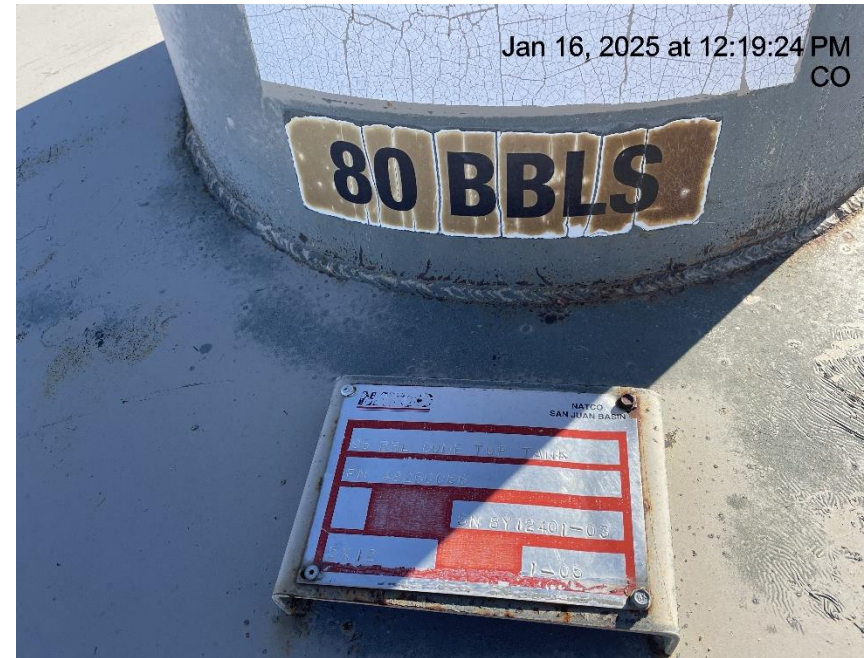
Photo # 9535 Capacity on tank label for blowdown tank is incorrect/does not comply with CECMC rules
