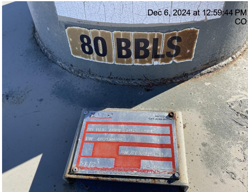
Photo # 2574 From inspection 708905205 conducted on 12/06/2024 Capacity on tank label for blowdown tank is incorrect/does not comply with CECMC rules
