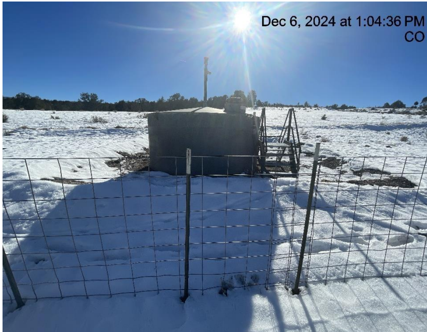
Photo # 2576 From inspection 708905205 conducted on 12/06/2024 Secondary containment insufficient/does not comply with CECMC rules
