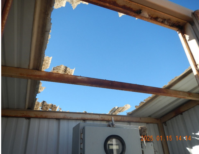
5. View of roof damage to remote gas meter shed.
