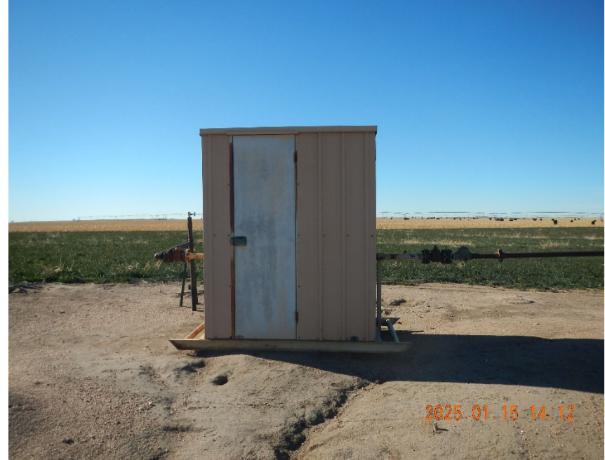
4. Gathering location overview. Note run off soil erosion around remote gas meter shed.
