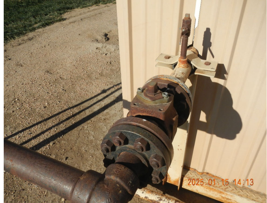
8. View of valve at remote meter shed. Both valves, Inlet and Outlet open at time of inspection.
