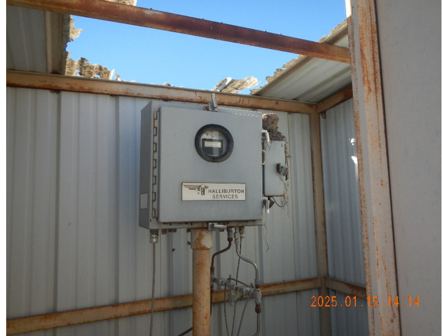
6. View of Gas Meter inside remote gas meter shed.
