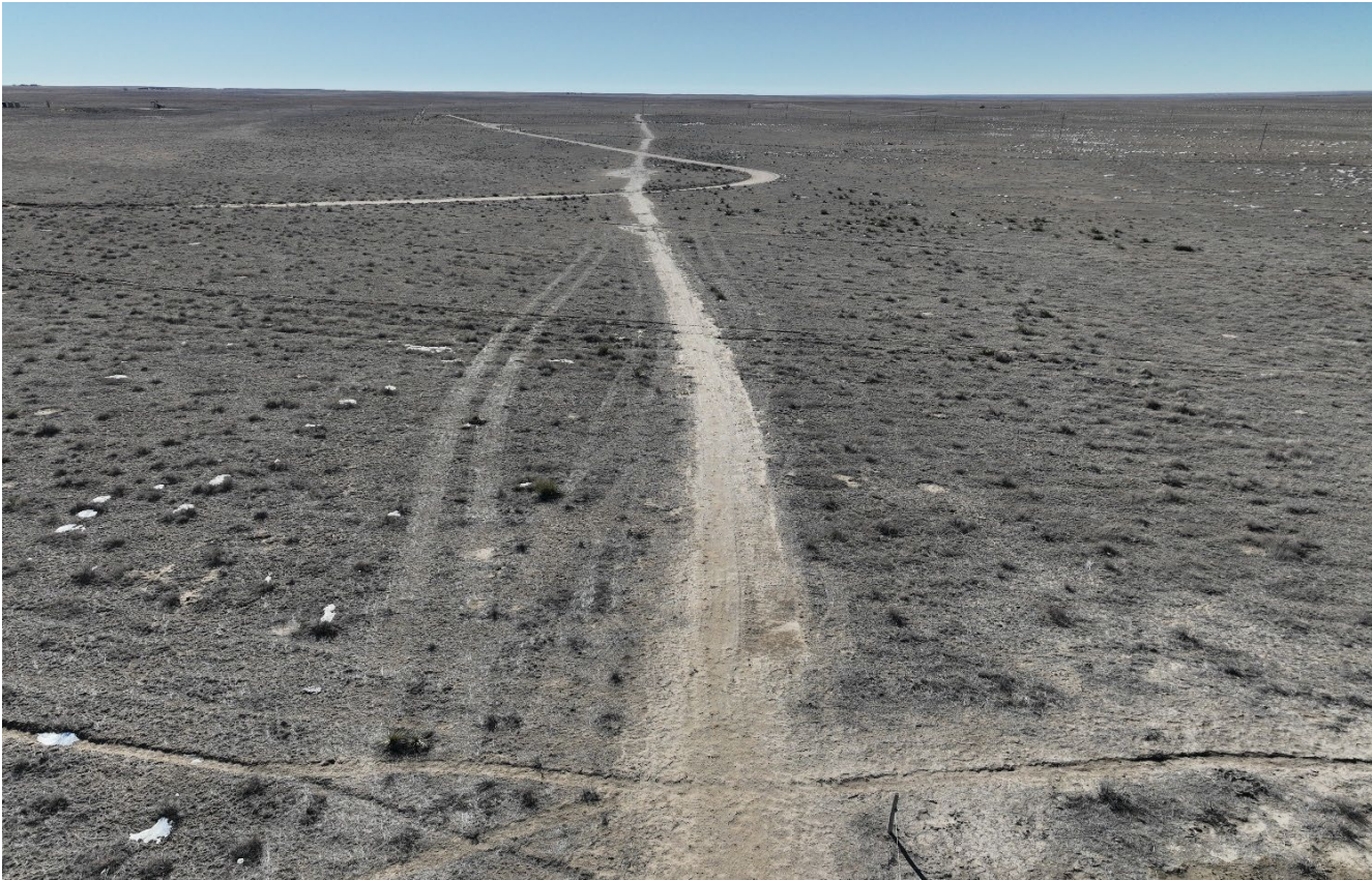
Photo 3. Facing south from the Dawson tank battery. A new flowline was installed and disturbance along the flowline must be reseeded and reclaimed before the upcoming growing season.
