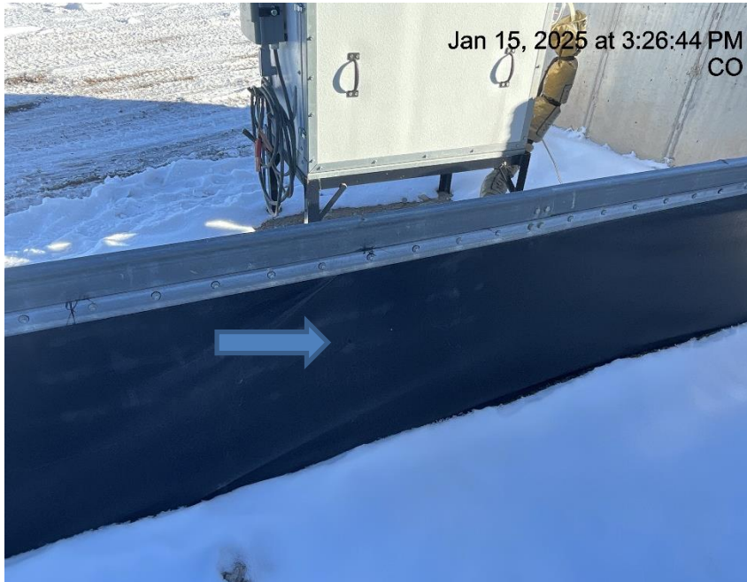
Photo # 9294 Hole in liner/liner needs maintenance
