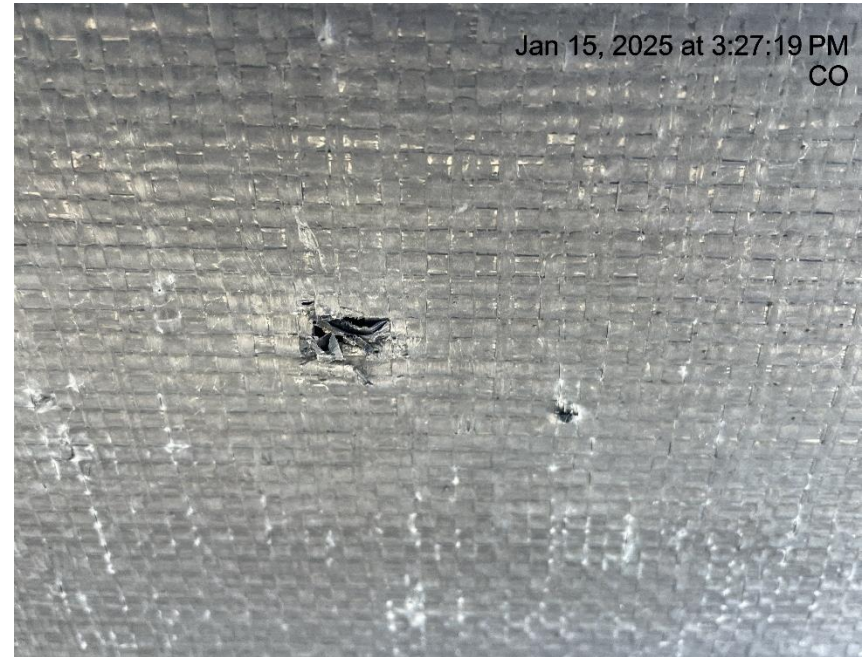
Photo # 9297 Hole in liner/liner needs maintenance
