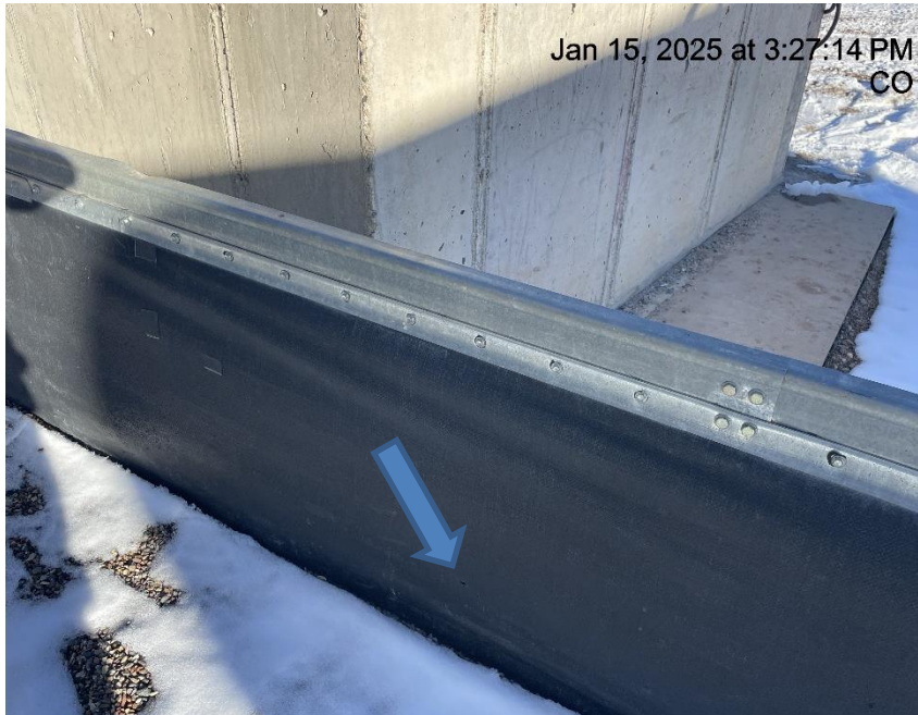
Photo # 9296 Hole in liner/liner needs maintenance
