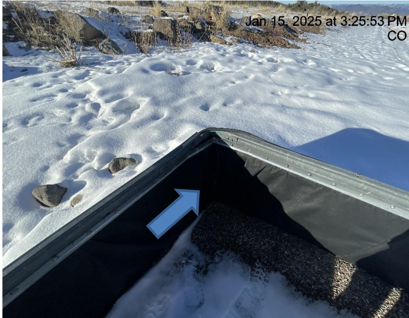
Photo # 9292 Hole in liner/liner needs maintenance
