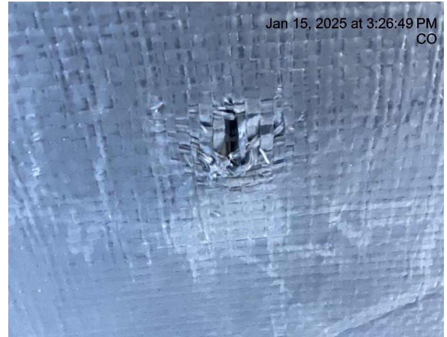
Photo # 9295 Hole in liner/liner needs maintenance
