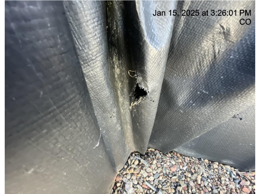
Photo # 9293 Hole in liner/liner needs maintenance
