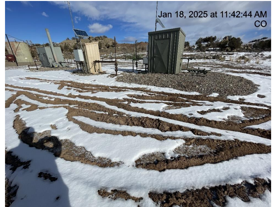
Photo # 71 Lack of stabilization/compaction
