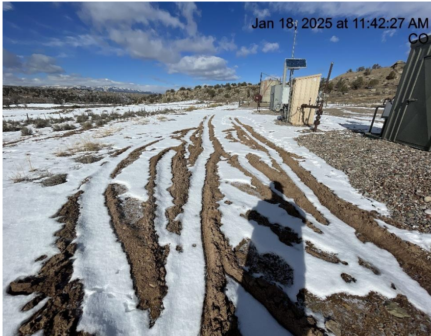
Photo # 70 Lack of stabilization/compaction
