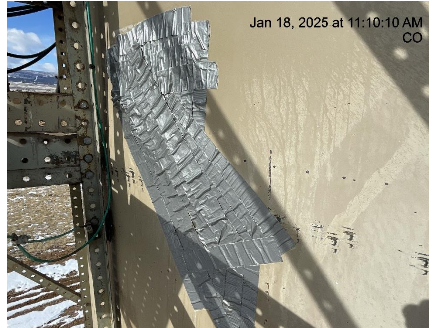
Photo # 9994 Possible tank integrity issue/tank appears to lack integrity
