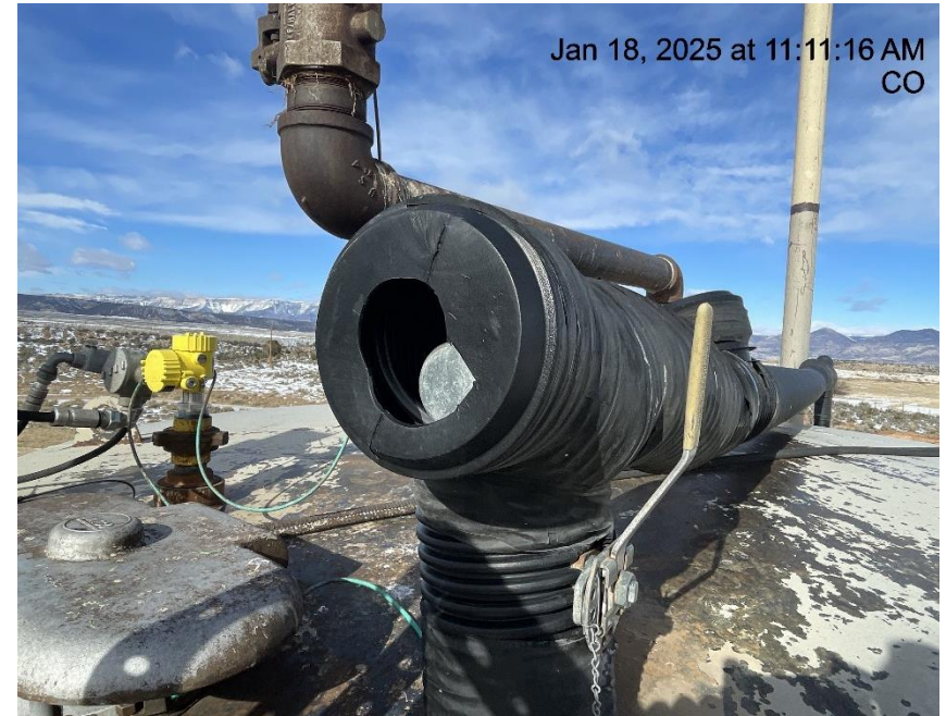
Photo # 9991 Flowline heating insulation damaged/wildlife hazard/available for entry by wildlife
