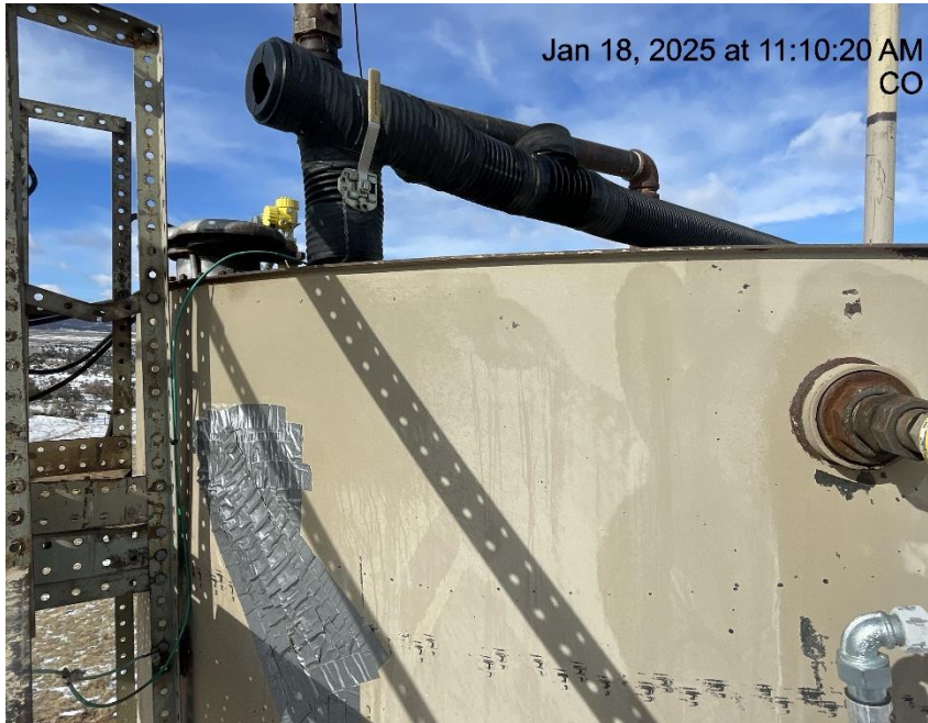
Photo # 9994 Possible tank integrity issue/tank appears to lack integrity
