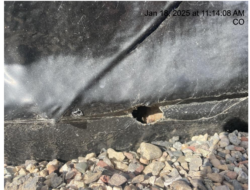
Photo # 9993 Hole in secondary containment liner/liner needs maintenance
