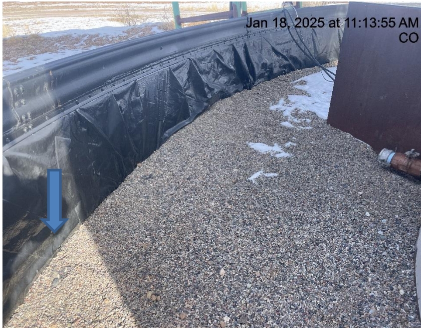
Photo # 9992 Hole in secondary containment liner/liner needs maintenance
