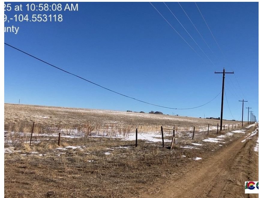
Pic 2 unable to access site due to low hanging utility cable.
