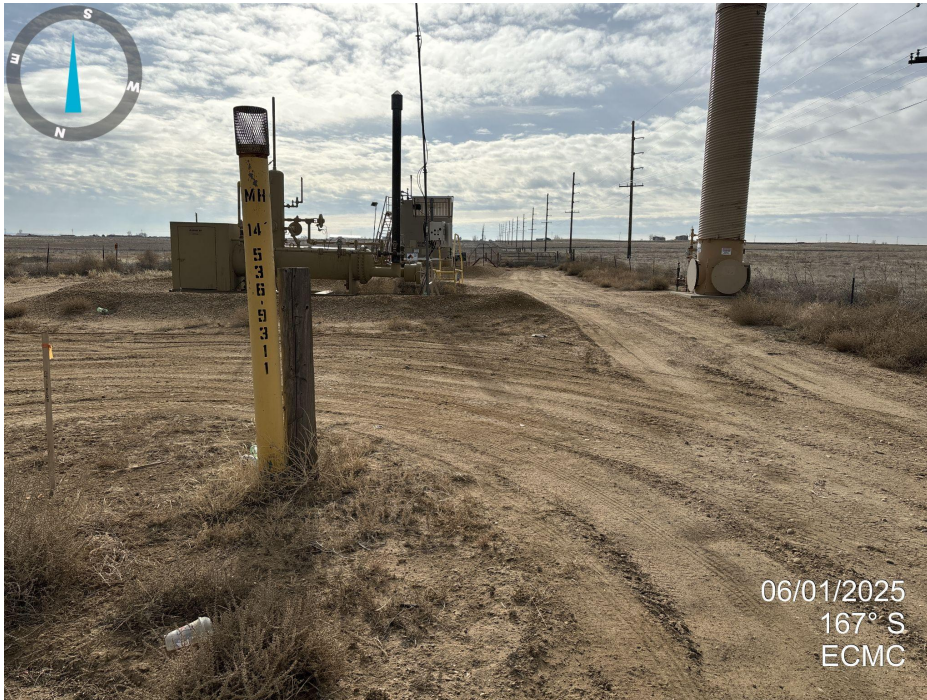
Photo 1. Looking south across tank battery. Bottles and other trash is present throughout the location.
