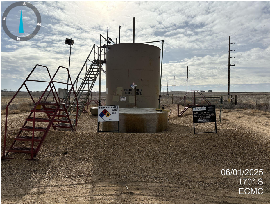
Photo 3. looking south at tank battery.
