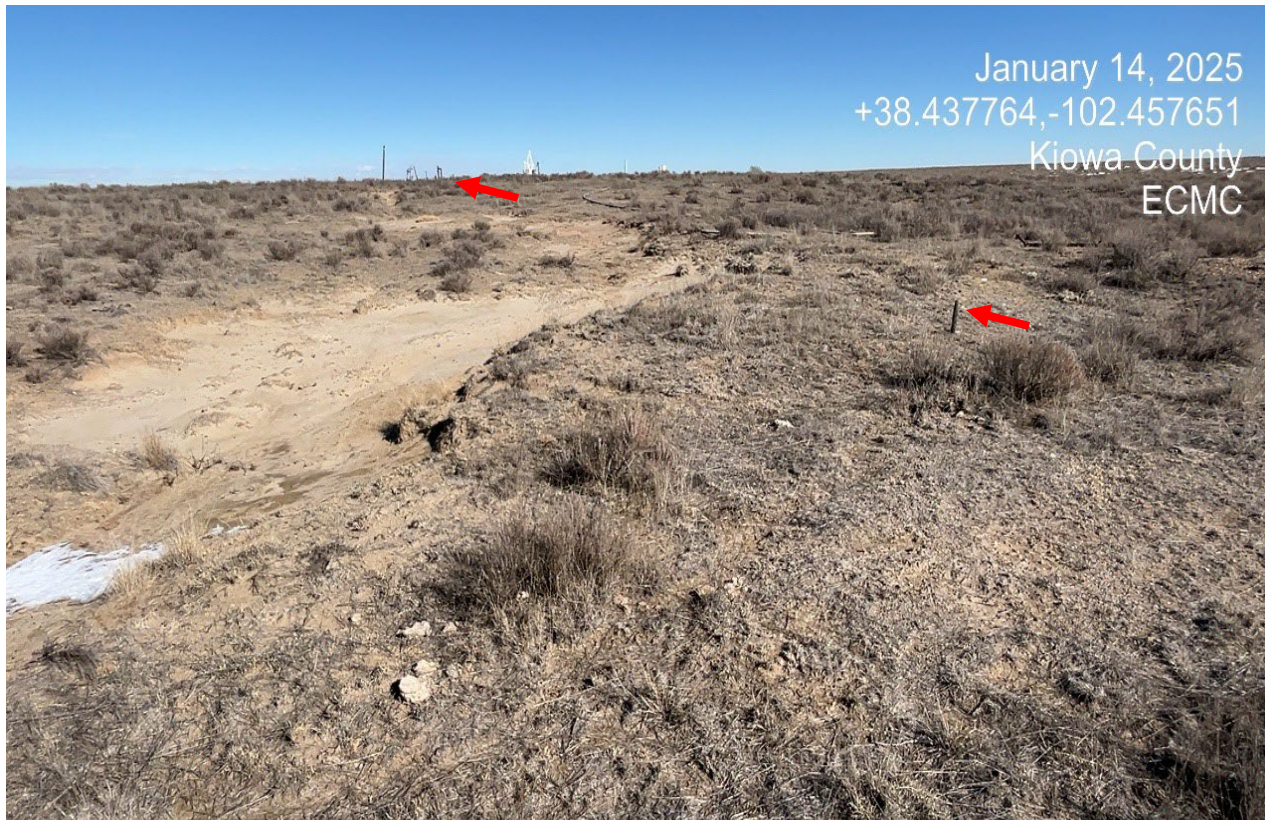
Photo 1. Facing northeast at the former wellsite. There appears to have been a historic impact where vegetation is not establishing. There are abandoned pipe risers shown at red arrows.
