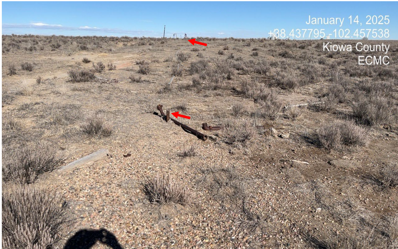
Photo 3. Facing northeast at the location. There are abandoned pipe risers shown at red arrows.
