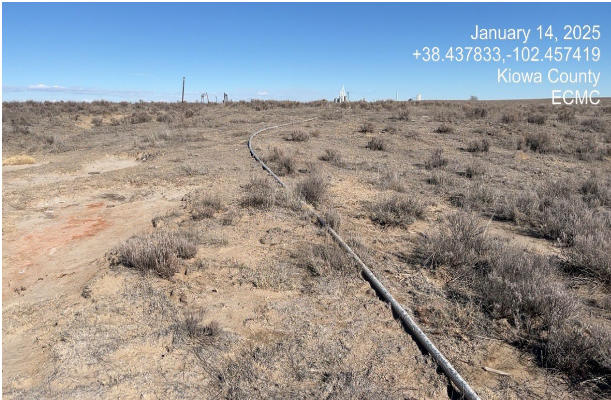
Photo 4. Facing northeast. There is a fiberglass pipe on the surface approximately 150' in length.
