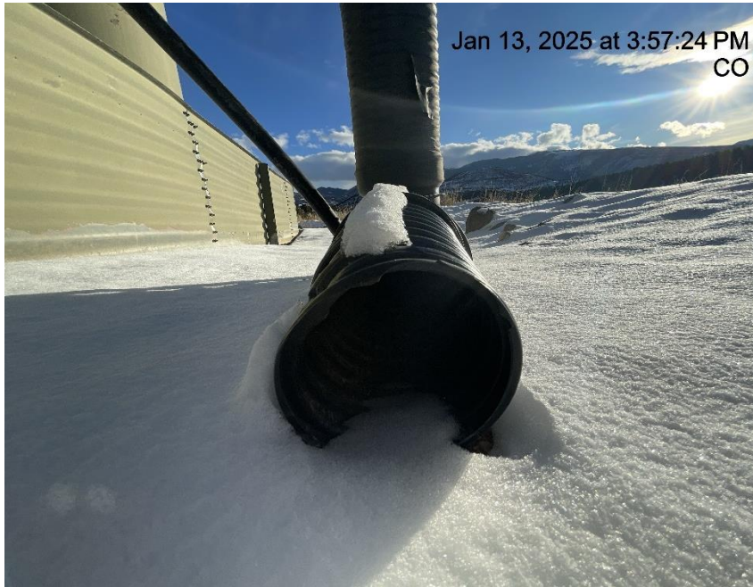
Photo # 8376 Flowline heating insulation open ended /wildlife hazard/available for entry by wildlife
