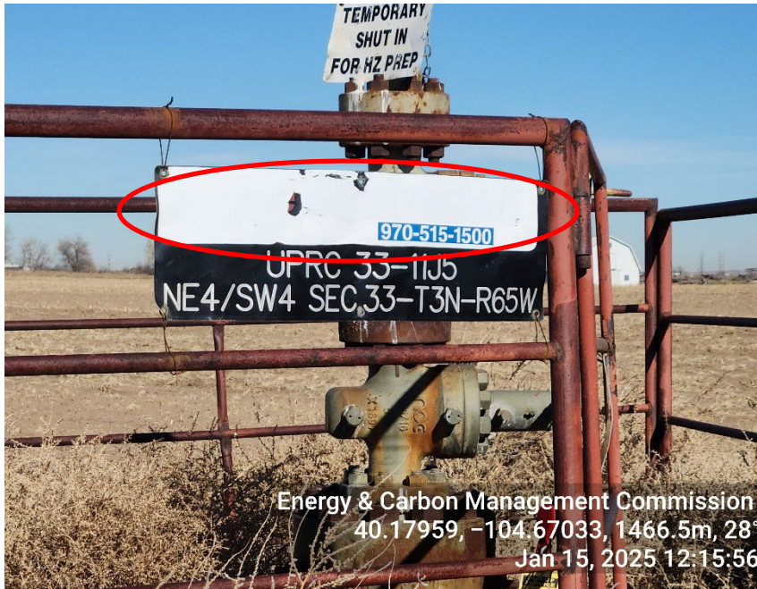
Photo 1: Wellhead Sign, operator name no longer legible
