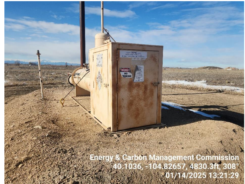
Photo 6 Horizontal Heated Separator.
