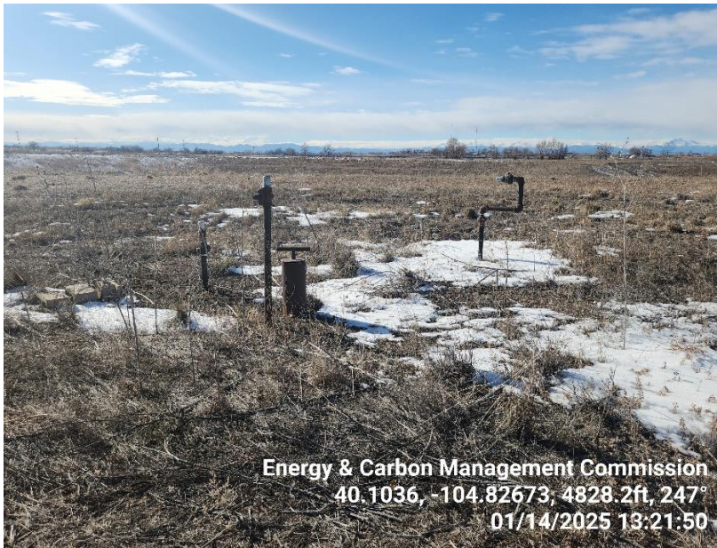
Photo 7 LOTO flow lines need to be re-tagged.
