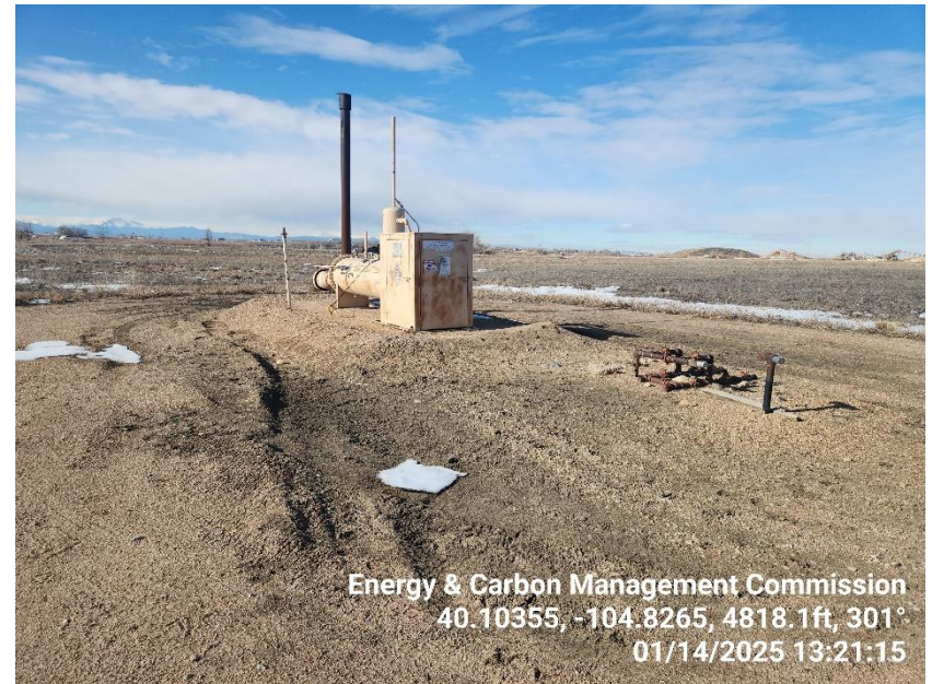
Photo 4 Horizontal Heated Separator & Flow line manifold.
