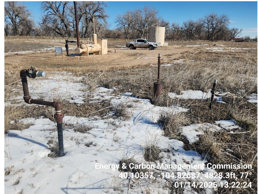
Photo 8 LOTO flow lines need to be re-tagged.
