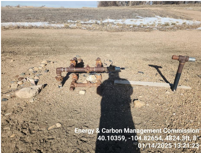
Photo 5 Flow line manifold.
