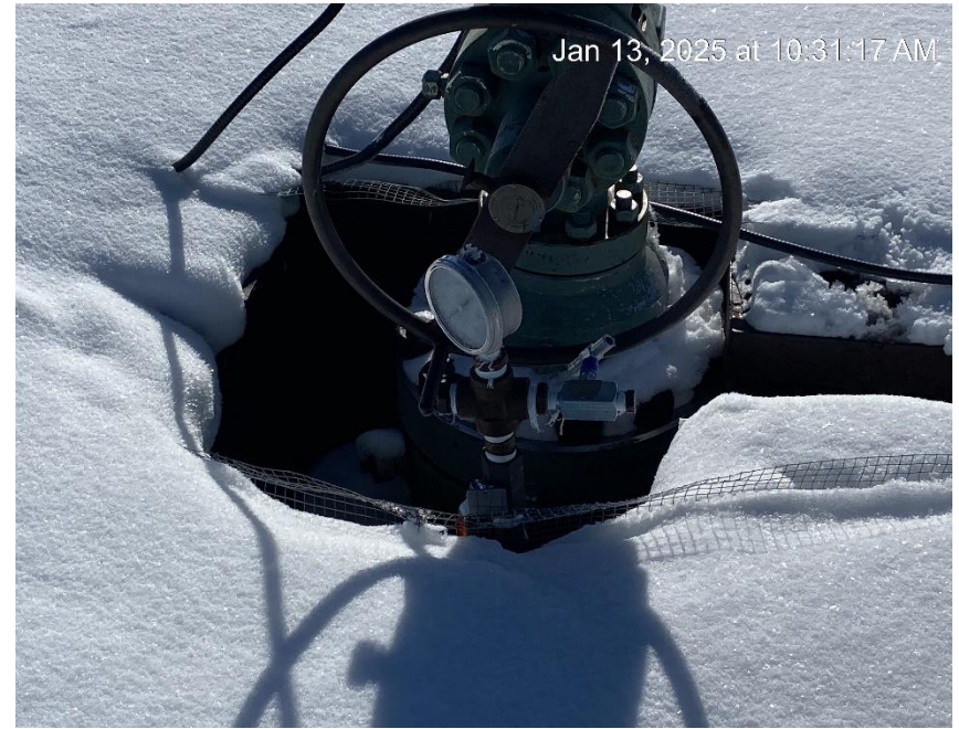
Cellar cover open around wellhead
