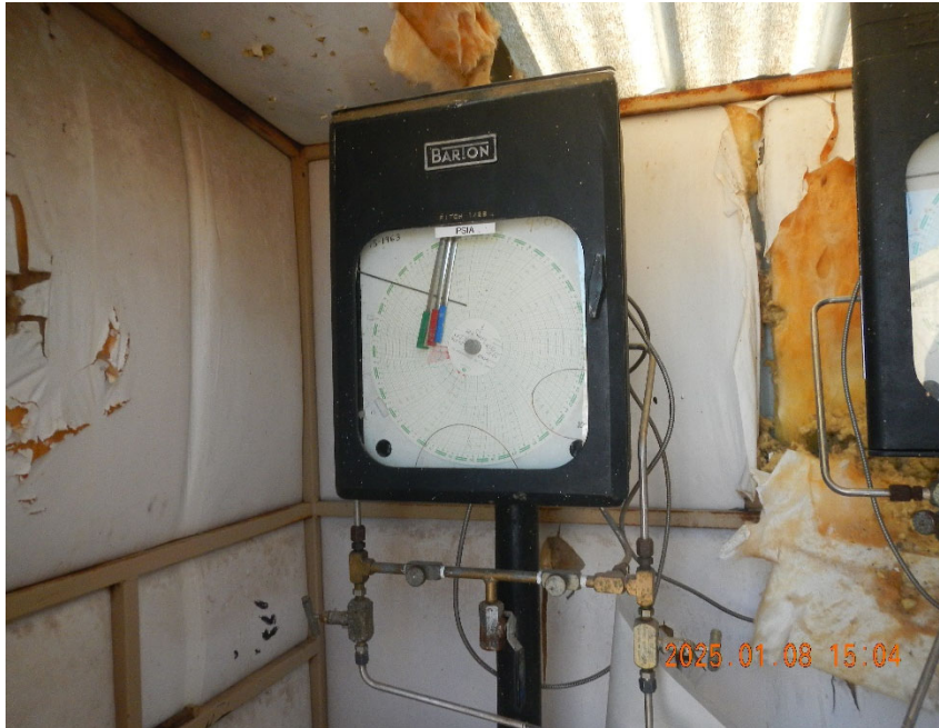
5. Gas meter inside meter shed.
