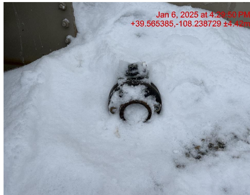
Photo # 2177 Open ended load line
