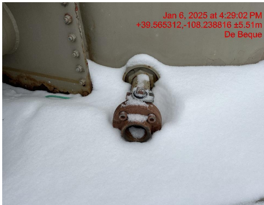
Photo # 2175 Open ended load line
