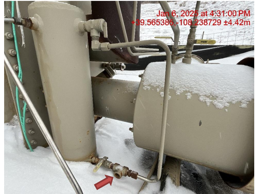
Photo # 2179 PRV vent line does not comply with CECMC pressure safety device rules
