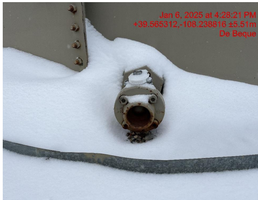
Photo # 2173 Open ended load line
