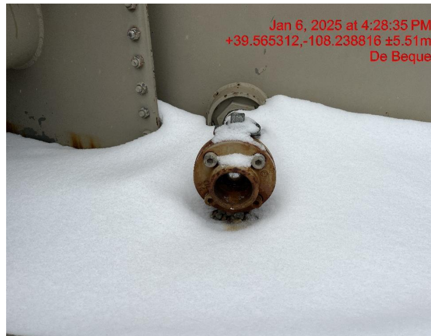
Photo # 2174 Open ended load line
