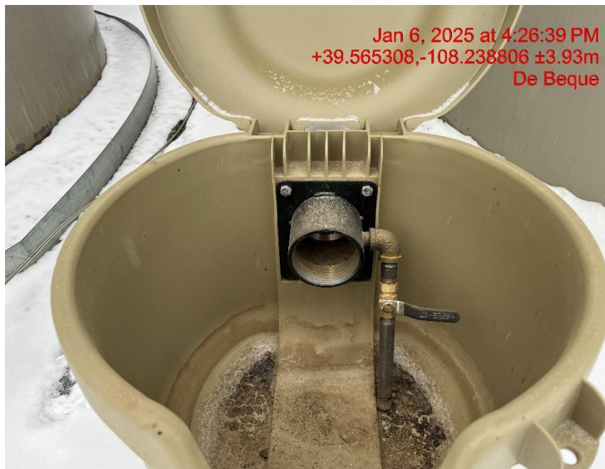
Photo # 2170 Open ended load line
