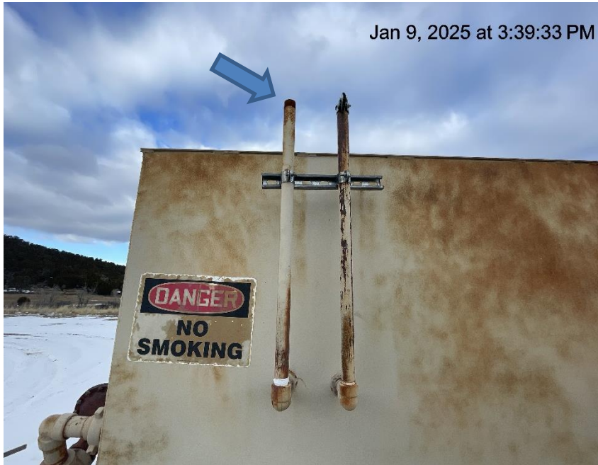
Photo # 8206 PRV vent line does not comply with CECMC pressure safety device rules
