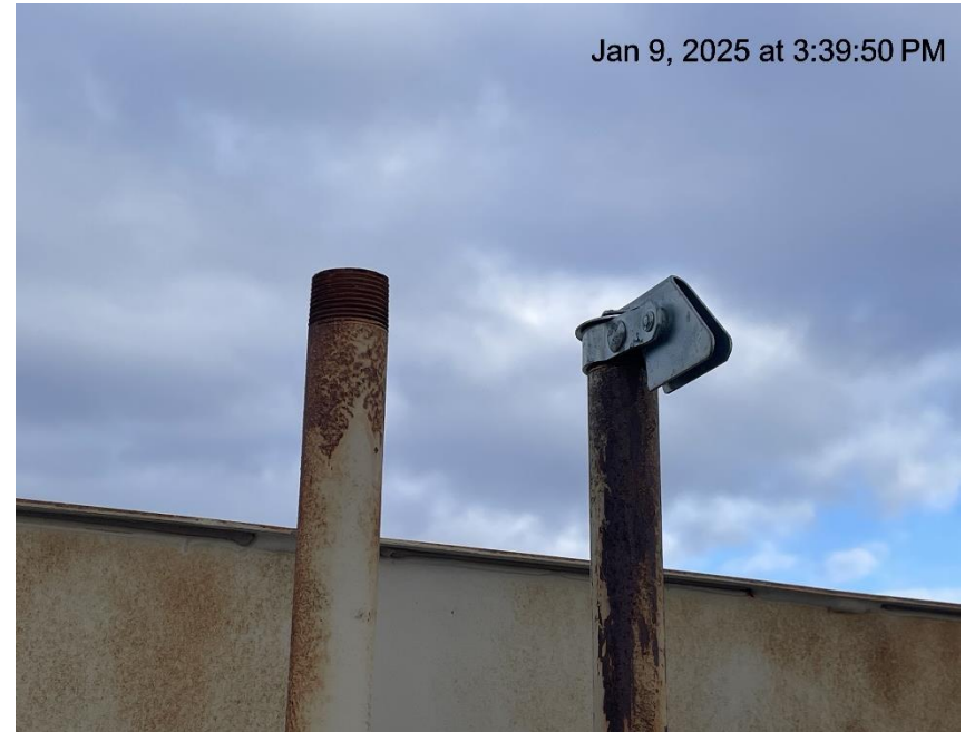
Photo # 8207 PRV vent line does not comply with CECMC pressure safety device rules
