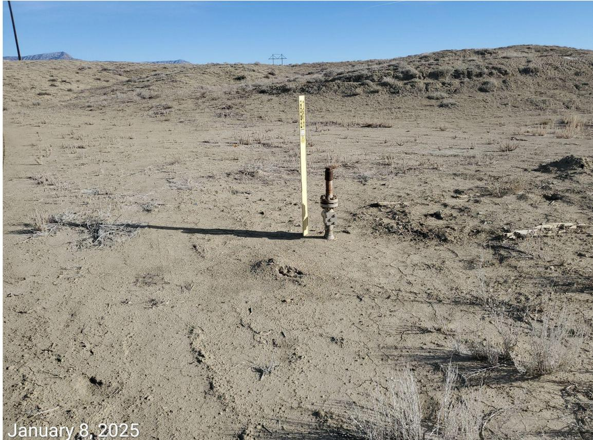
**Photo 4:** Photo shows surface equipment (riser) remaining on the north end of the Location.
