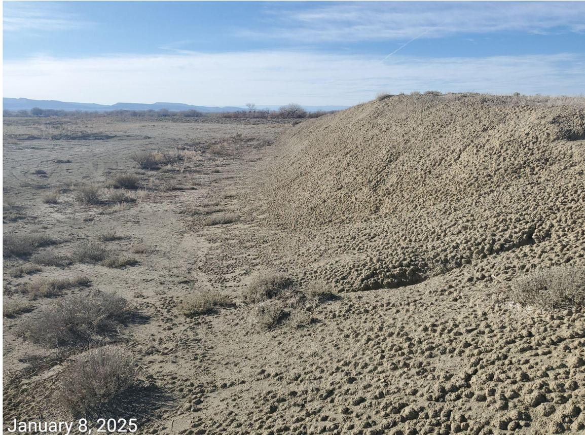
**Photo 6:** Photo taken from the northeast corner of the Location, facing west. Photo shows the cut slopes; Location has not been decompacted, recontoured/regraded and reclaimed
