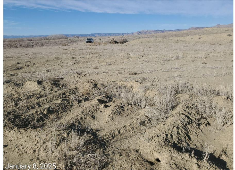
**Photo 1:** Photos 1-2 taken from the south end of the Location. Photos provide an overview of the Location from west, northwest, northeast to east. Photos show final reclamation has not been performed in accordance with 1004 requirements- Location/Road has not been decompacted, recontoured/regraded and reclaimed; Undesirable and Noxious Plant Species (Halogeton) observed established throughout the Location disturbance.
