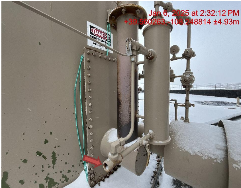
Photo # 2078 PRV vent line does not comply with CECMC pressure safety device rules
