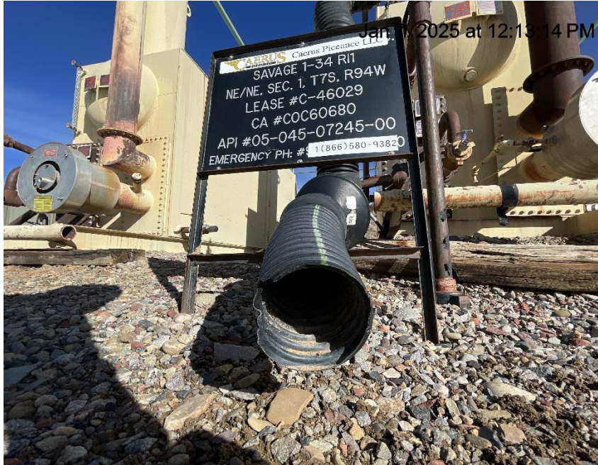
Photo # 7207 Flowline heating insulation open ended /wildlife hazard/available for entry by wildlife
