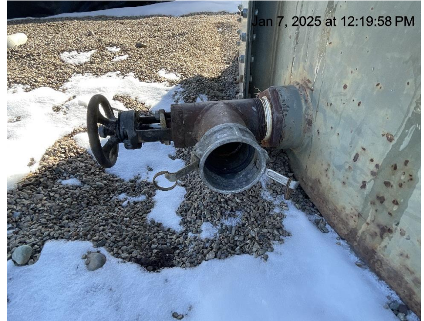
Photo # 7208 Open ended load line
