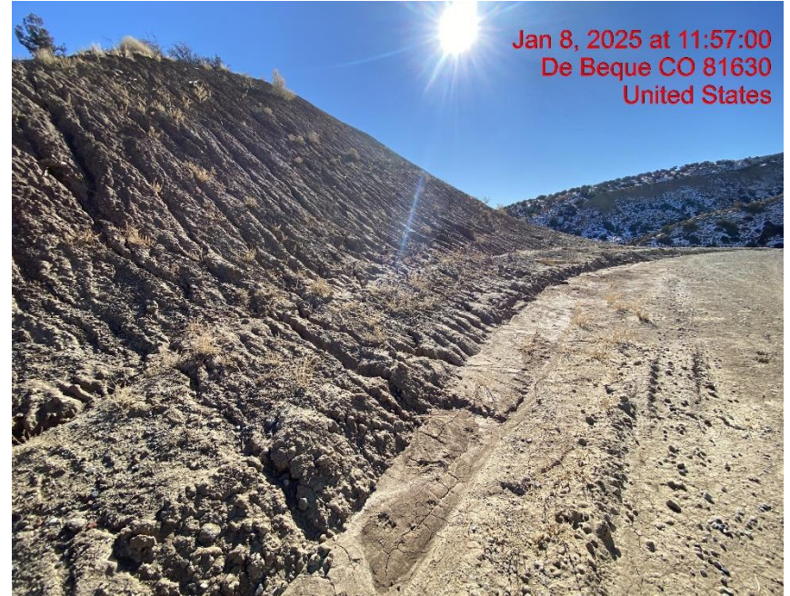
Insufficient Erosion Controls/Ditch Needs Maintenance – Photo #05846
