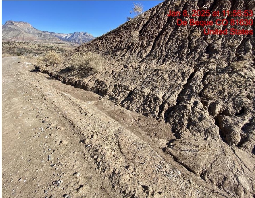
Insufficient Erosion Controls/Ditch Needs Maintenance – Photo #05845
