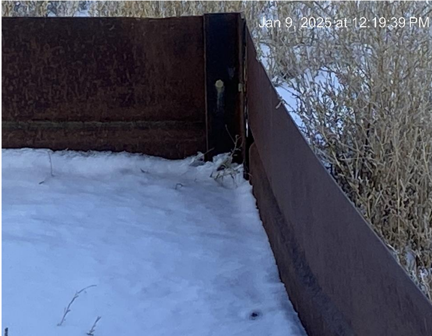
Gap in containment connection
