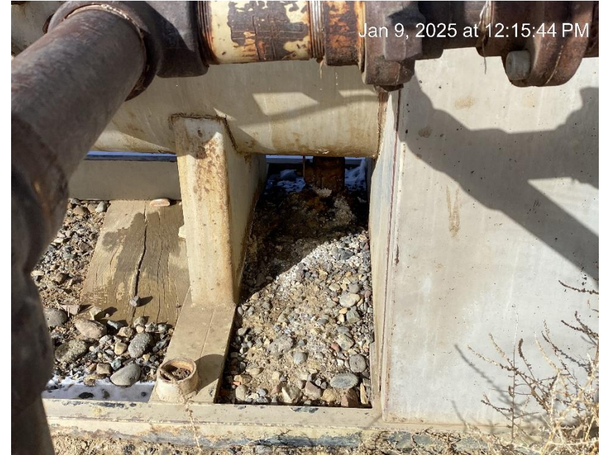
Leaking equipment. Staining.
