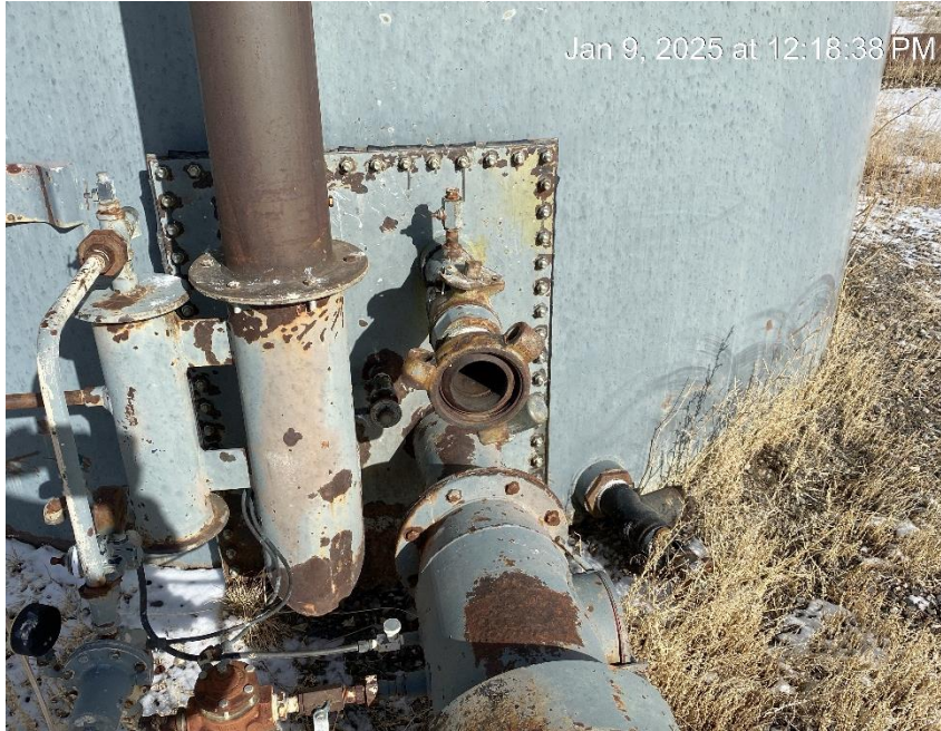
Open end tank valve. Open to wildlife.
