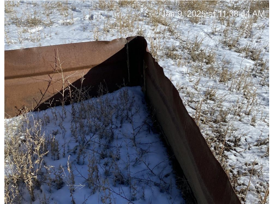
Damaged tank containment
