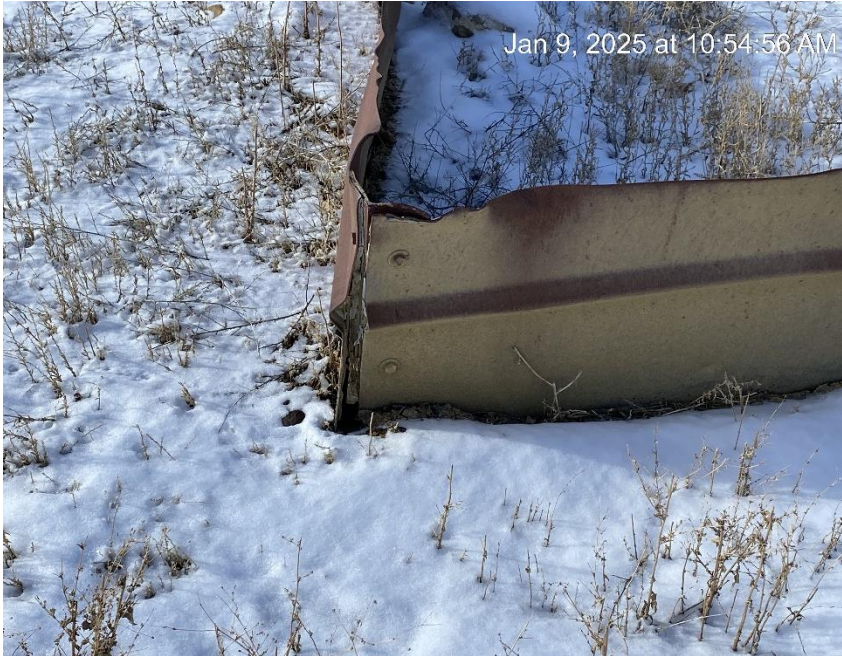
Damaged tank containment
