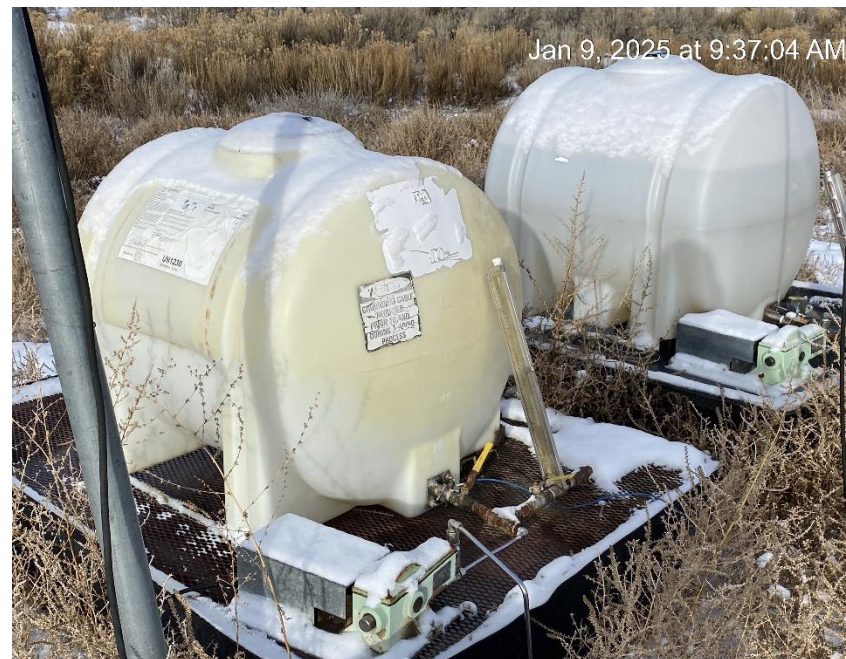
Faded chemical tank labels
