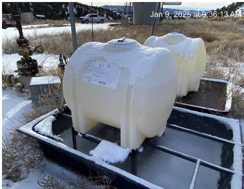
Faded chemical tank labels
