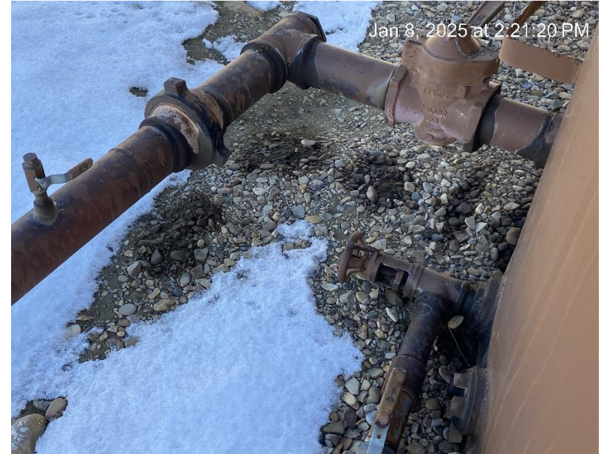
Leaking equipment. Staining.
