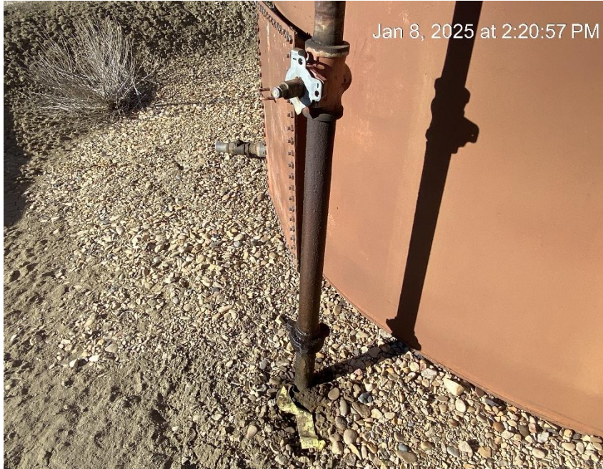
Leaking equipment. Staining.
