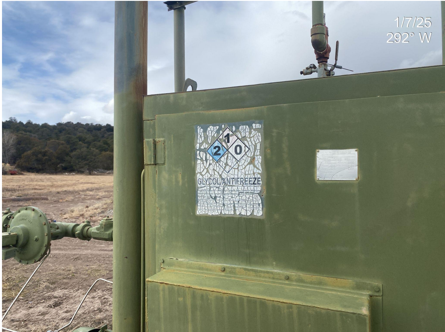
Photo 2. Label at separator has deteriorated and is no longer legible.
