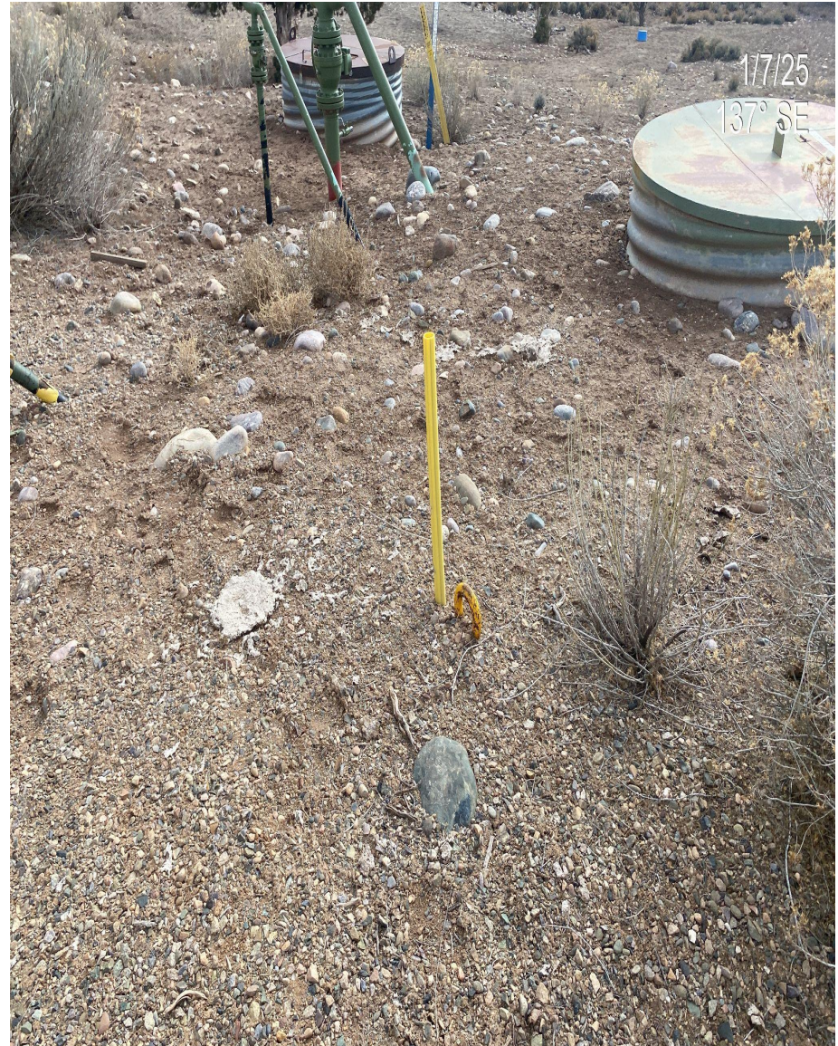
Photo 2. View of marked guylines anchors on location.
