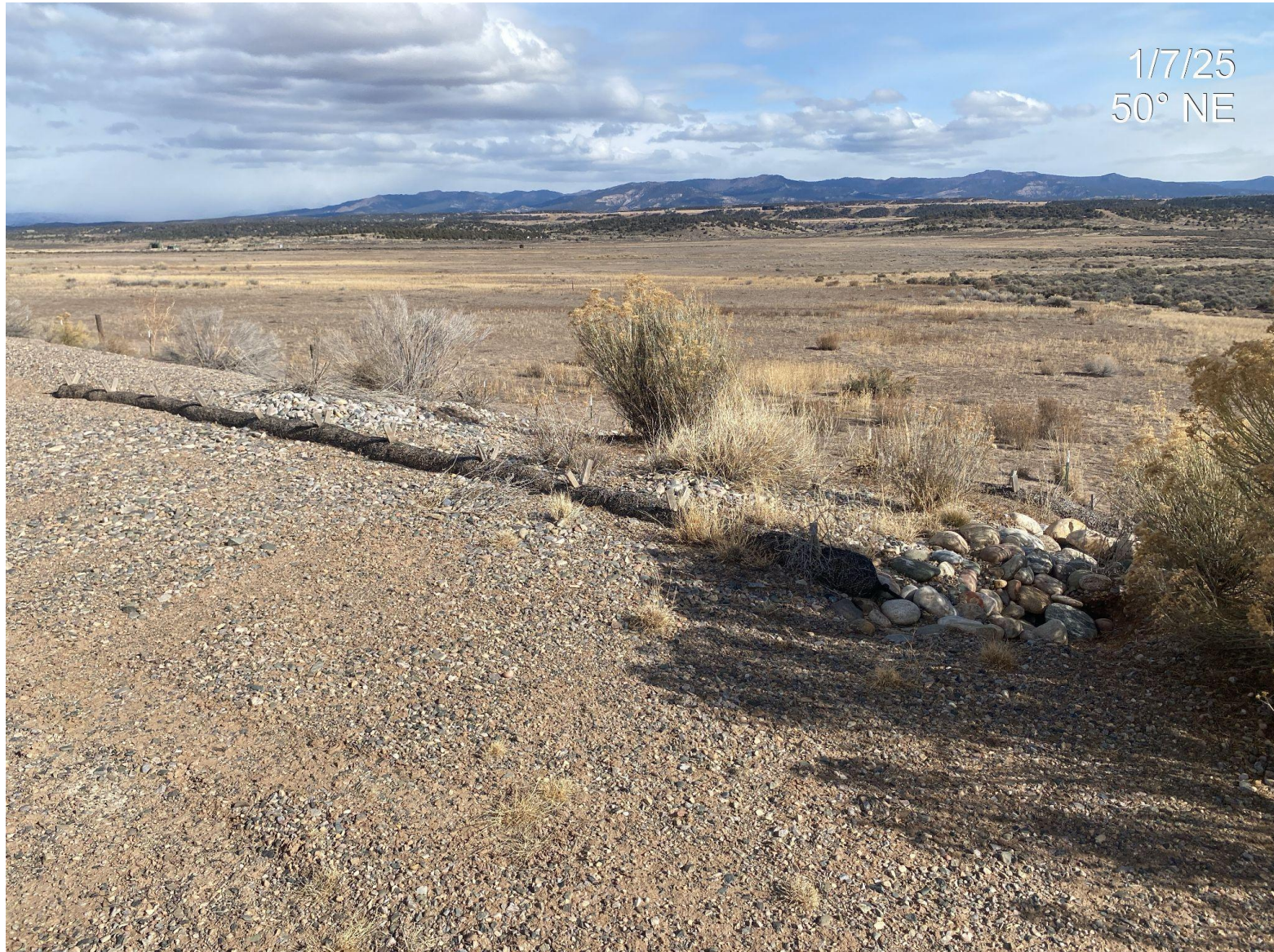
Photo 3. Stormwater BMPs have been installed in the eastern portion of the disturbance.
