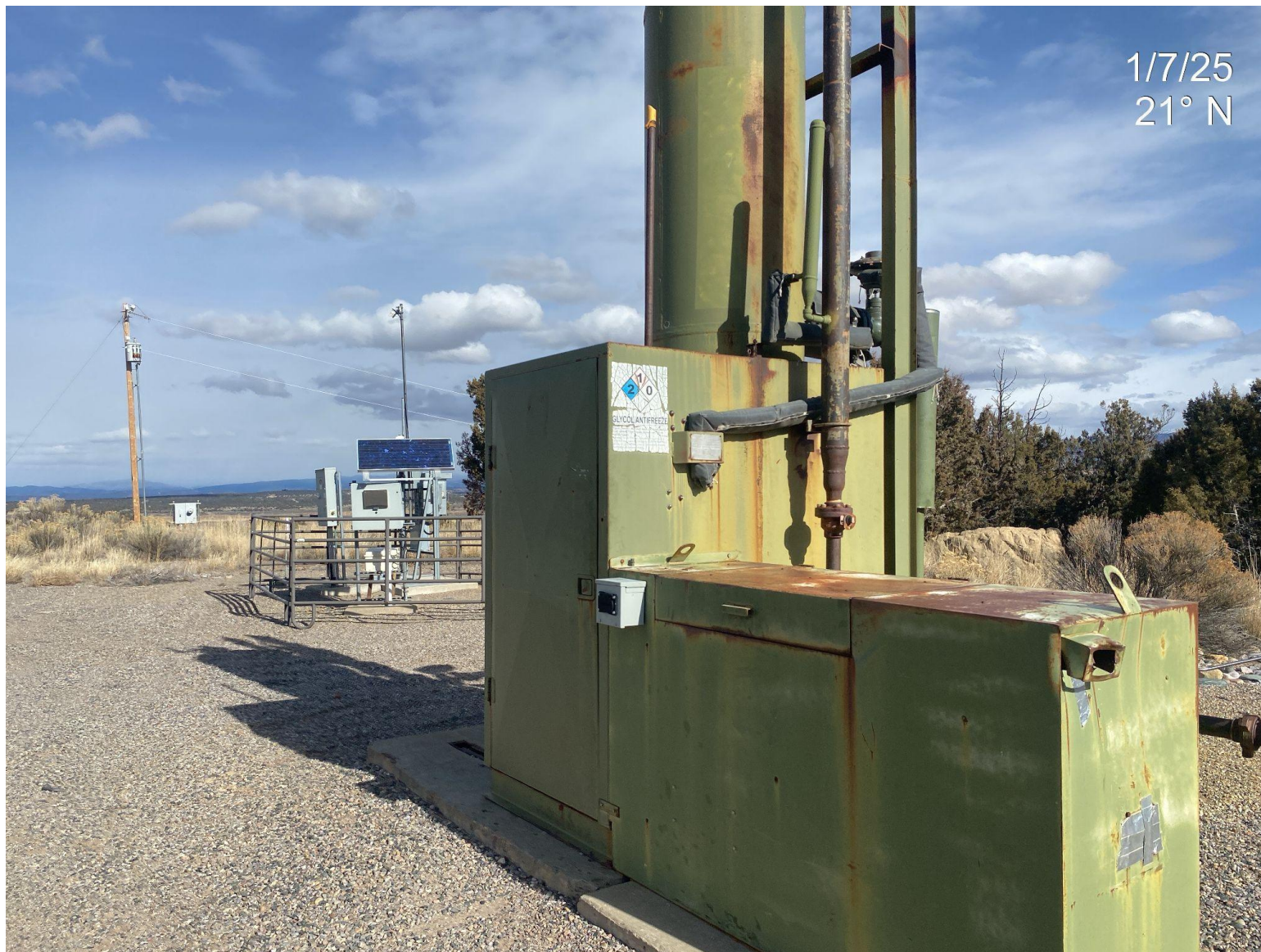
Photo 5. Label at separator is starting to deteriorate but still legible, future maintenance is advised.
