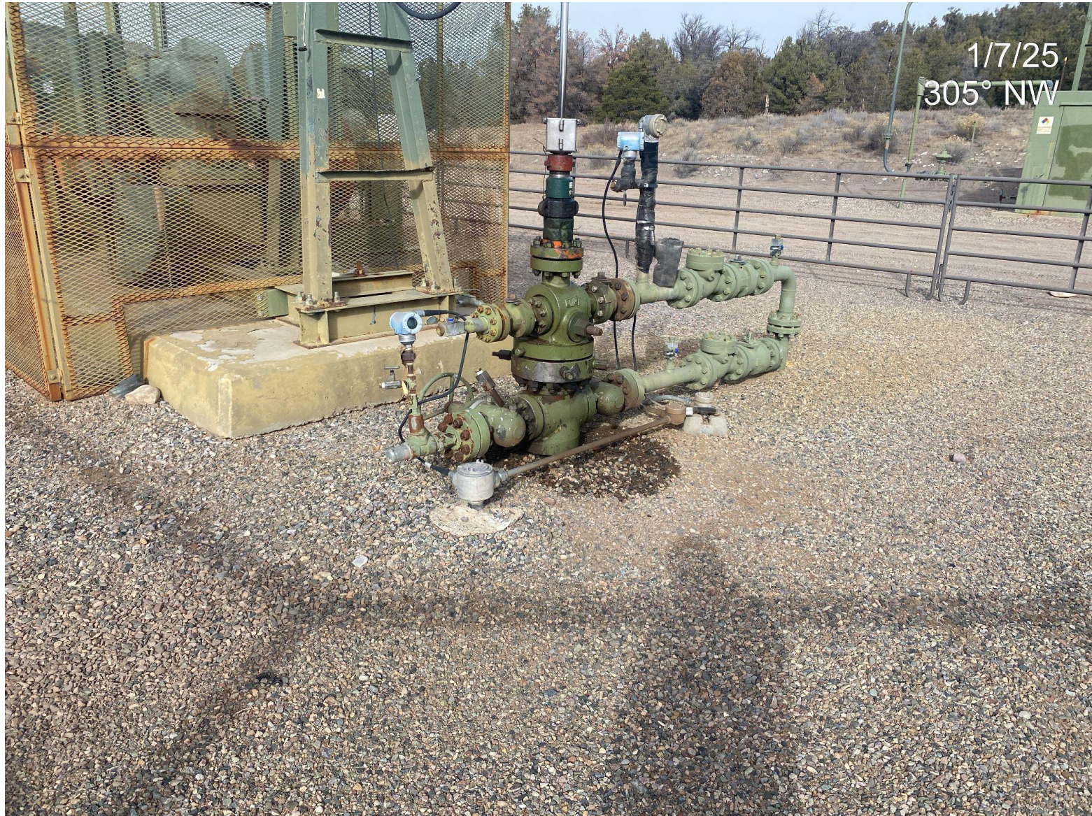
Photo 4. Impacted surface material observed at well head B1.
