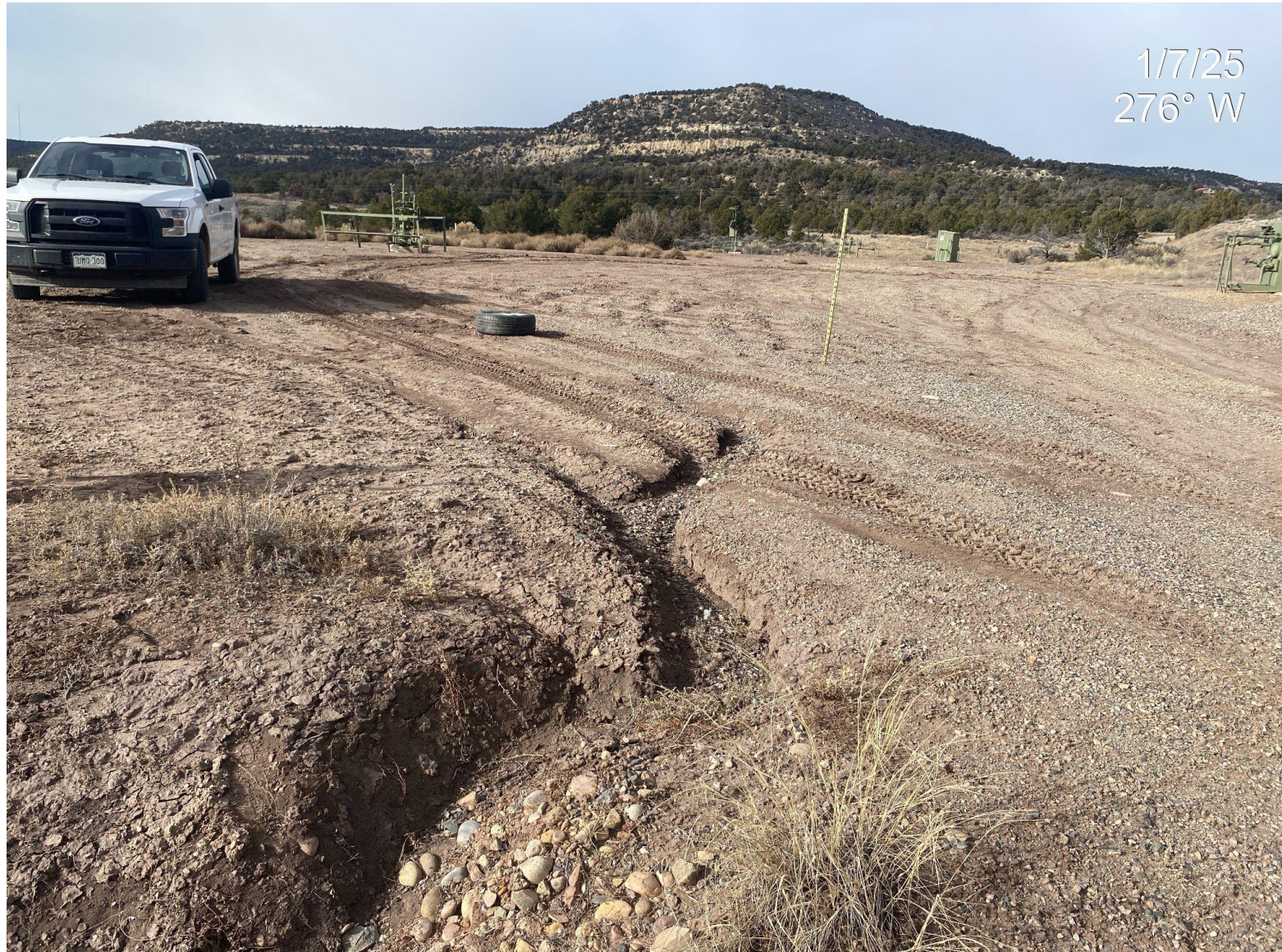
Photo 2. Gully erosion forming at location access point.
