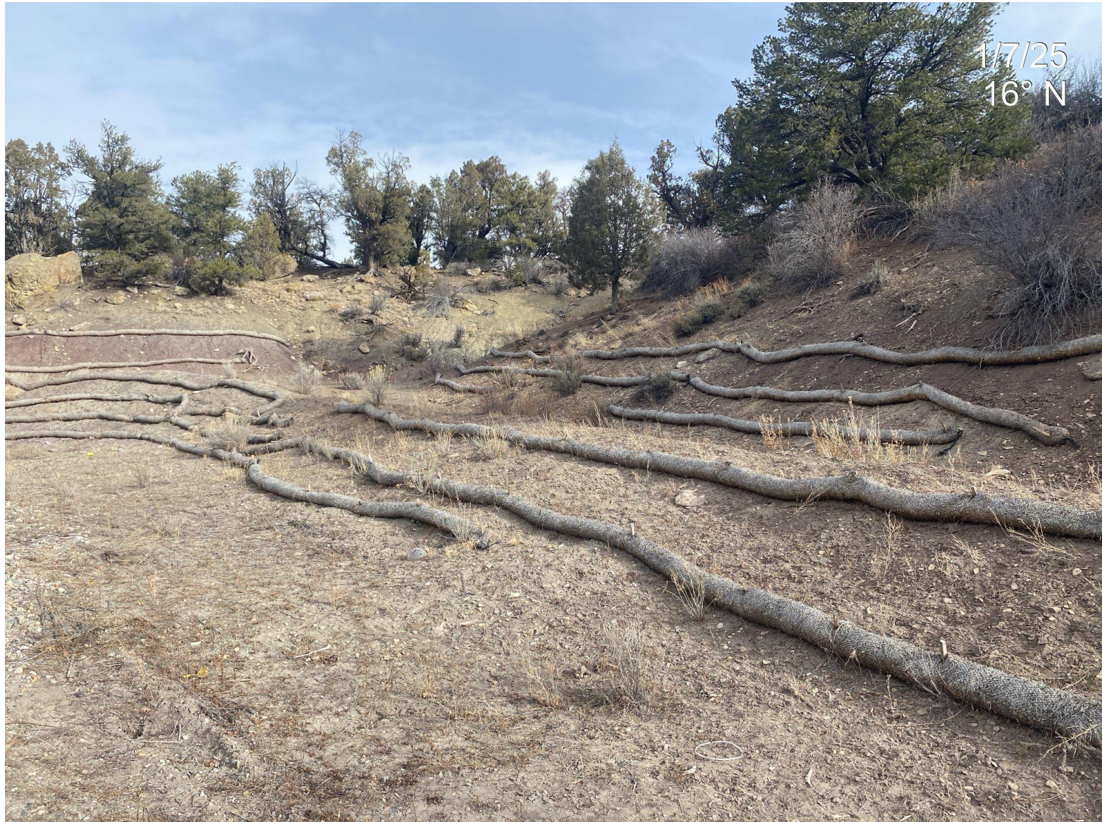
Photo 3. Stormwater BMPs installed in the eastern cutslope area. Vegetation is progressing in this area.
