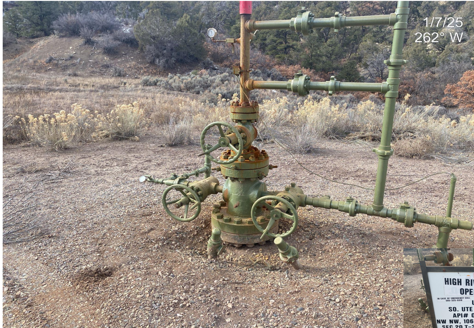
Photo 1. View of wellhead assembly.
