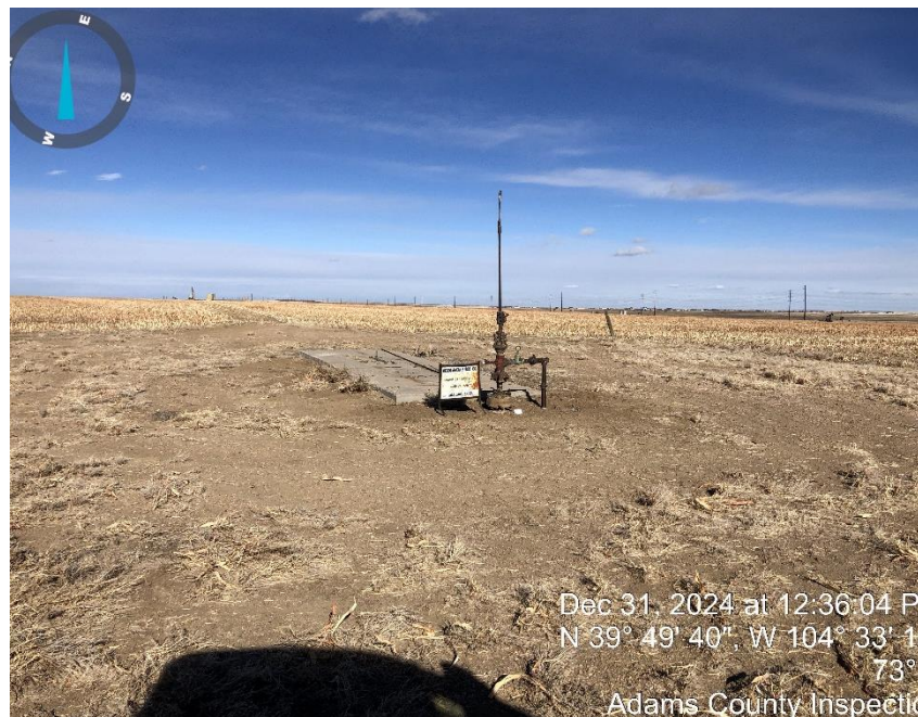
Photo #1 Well head.
