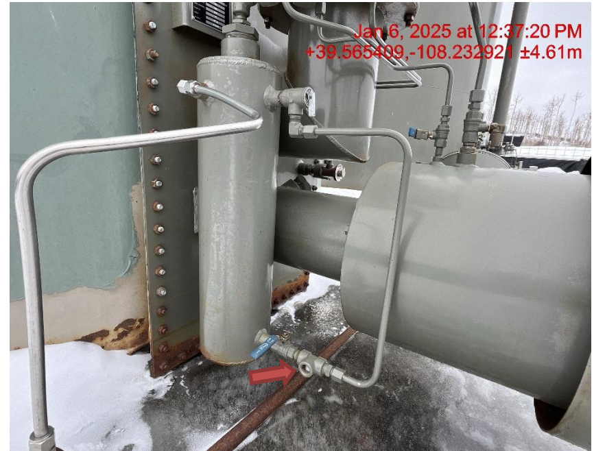
Photo # 1983 PRV vent line does not comply with CECMC pressure safety device rules
