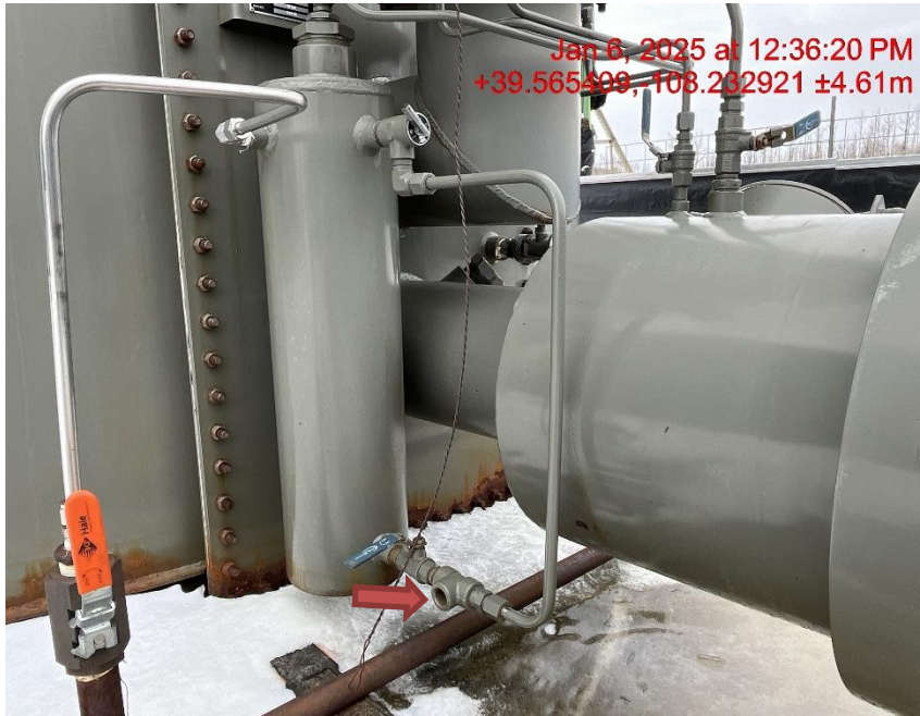
Photo # 1982 PRV vent line does not comply with CECMC pressure safety device rules
