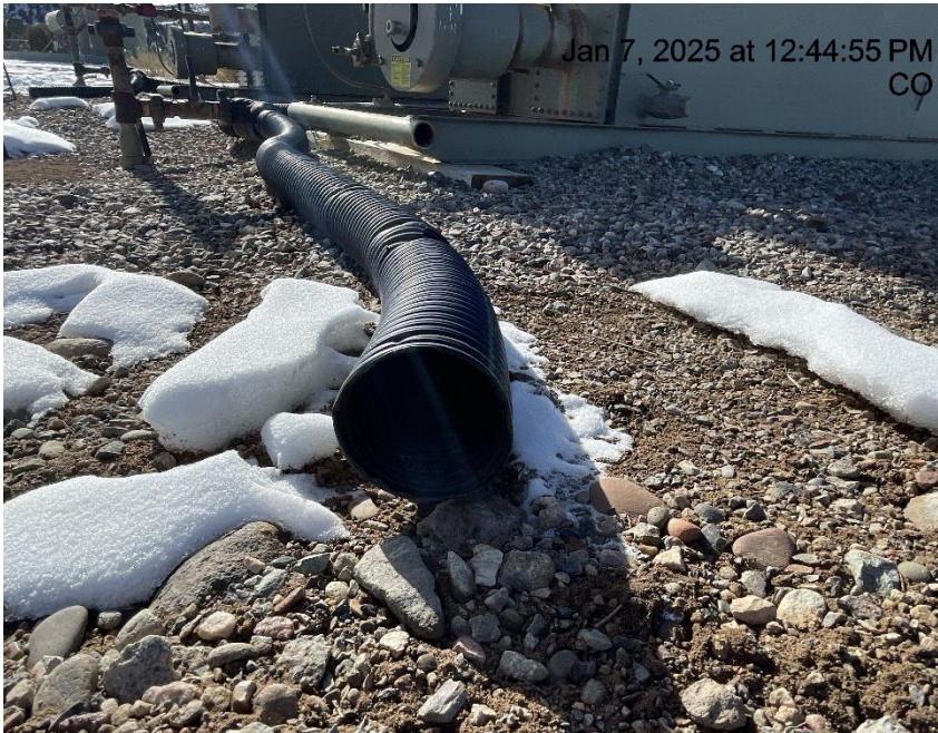
Photo # 7338 Flowline heating insulation open ended /wildlife hazard/available for entry by wildlife
