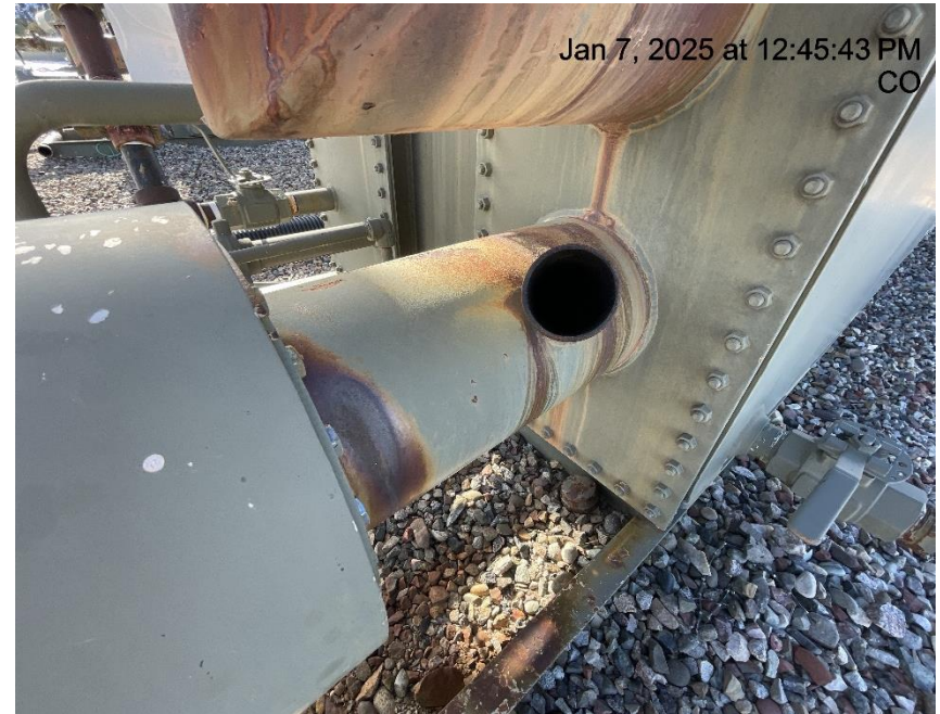
Photo # 7339 Burner tube missing cap/open ended/wildlife hazard/available for entry by wildlife
