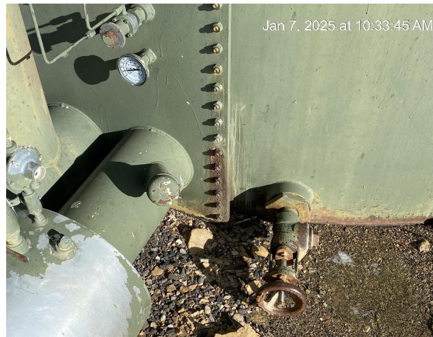
Hatch leak
