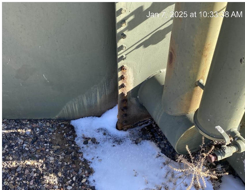
Hatch leak
