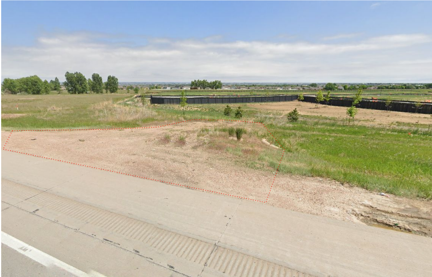
Photo 3. Google Maps imagery (reportedly from May 2024) illustrating that the former tank battery access road off of US 34 does not appear to have been reclaimed with evidence of road base material, culvert and contouring/grading that is not reflective of the adjacent areas.
