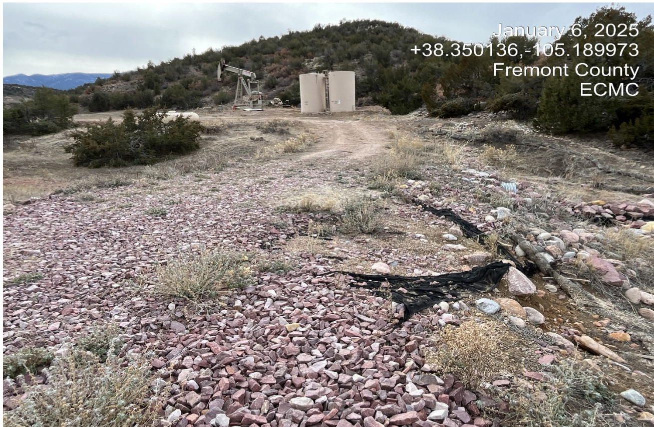
Photo 1. Facing toward the drainage crossing which has been washed out and has not been repaired. Previous corrective action was not completed.
