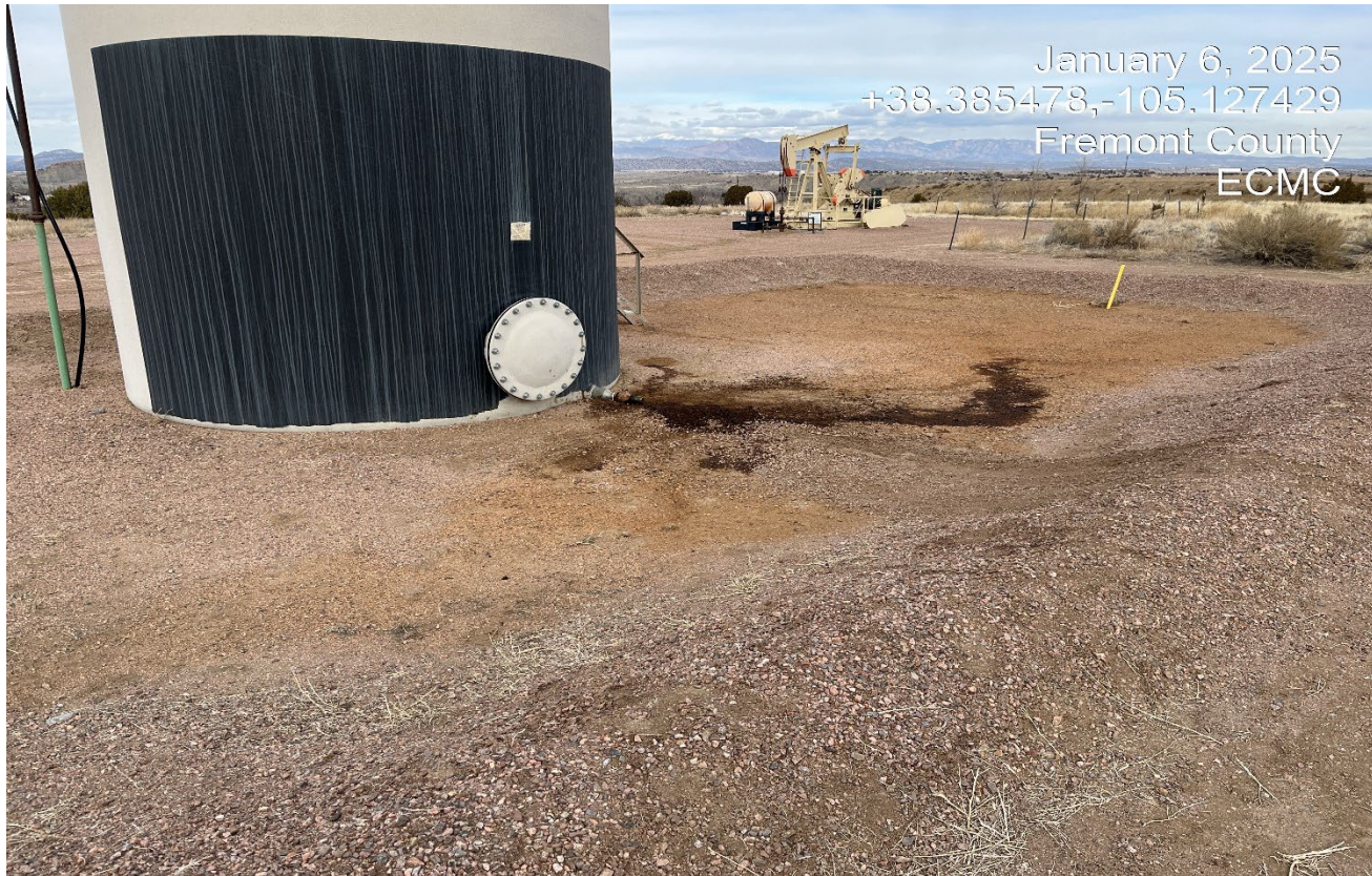
Photo 2. A spill occurred at the tank and impacted soils must be cleaned up.
