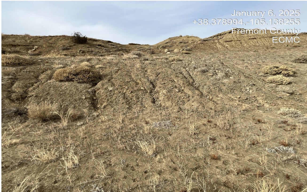
Photo 7. Facing toward the cut slope. There are riling erosion along the cut slope which is not stabilized. Previous CA was not completed.
