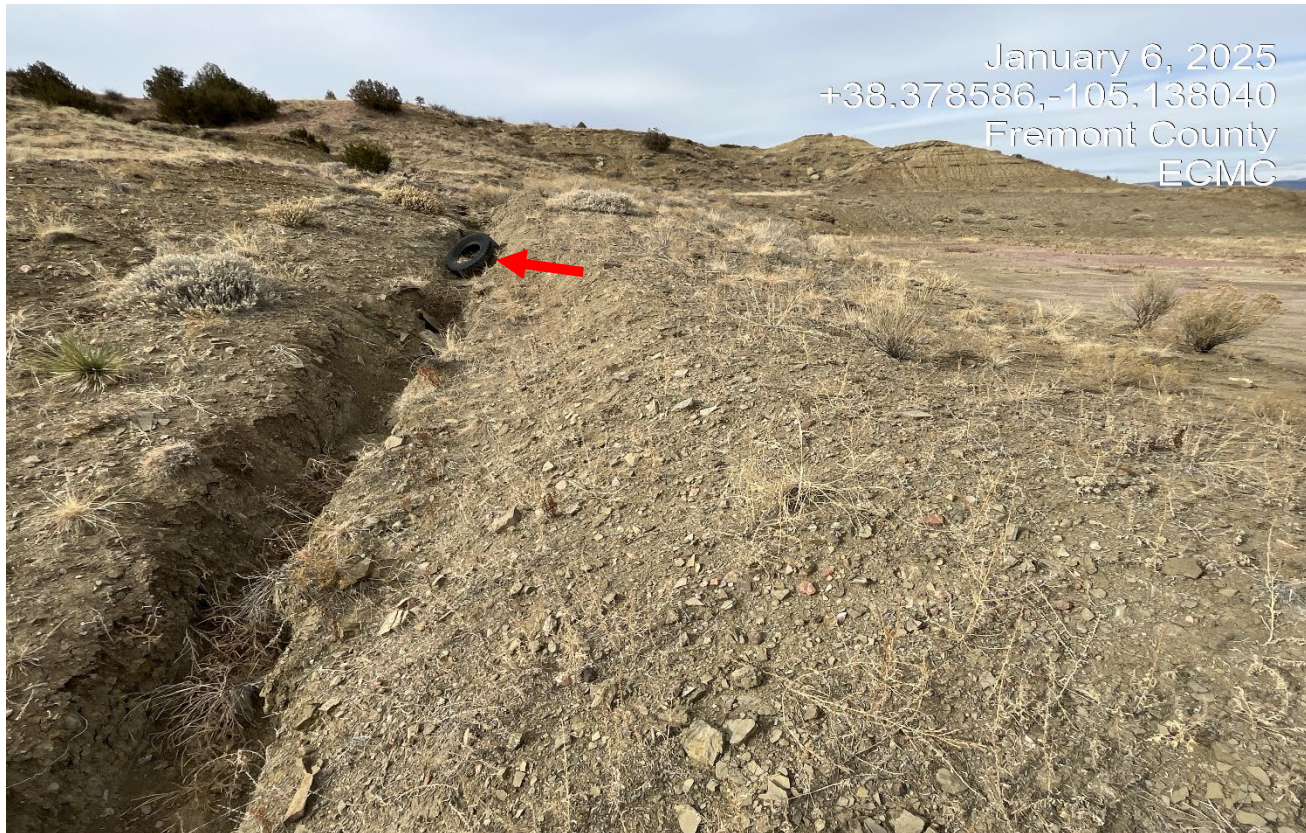
Photo 6. Facing southwest at the south side of the location. There is an erosion channel shown at red arrow which will need to be repaired and stabilized.
