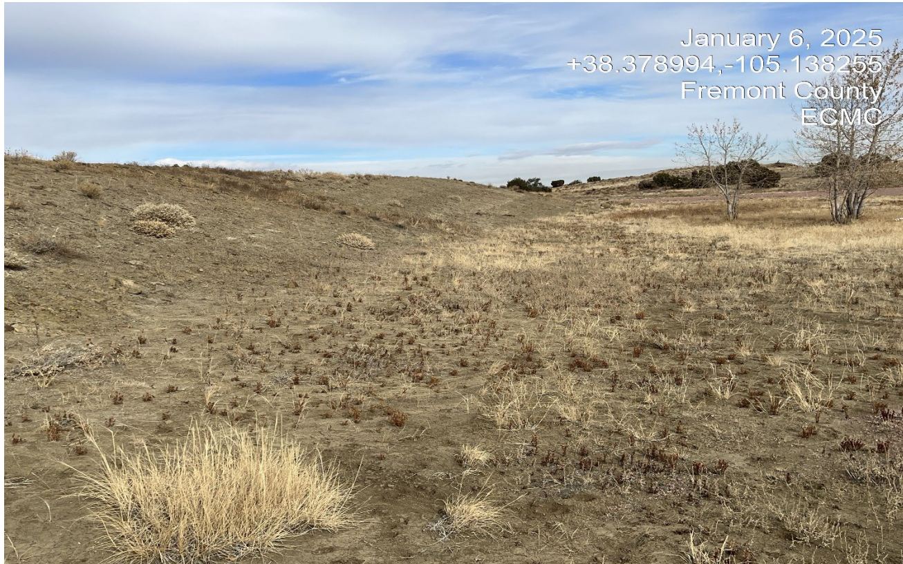
Photo 8. Facing northwest along the cut slope. There cut slope is not stabilized.
