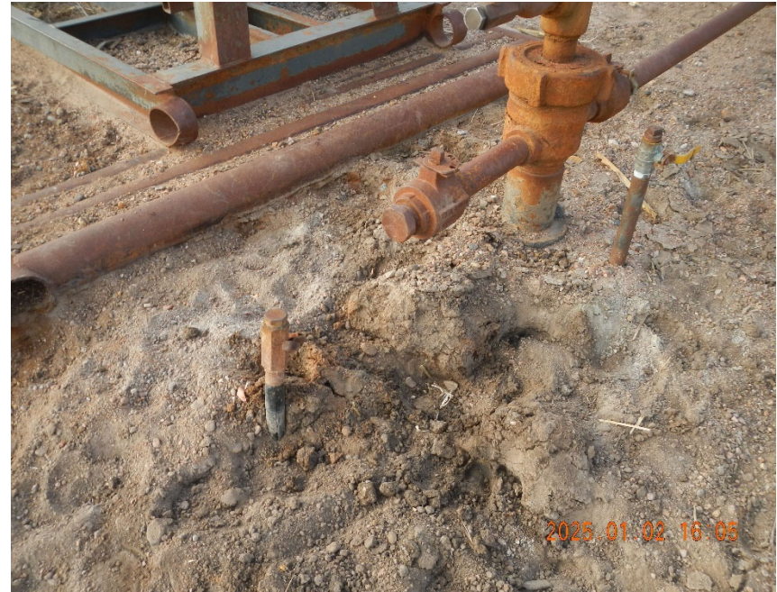
2. View of wellhead. Note water leg disconnected to resolve previously identified water leak. CA complete.
