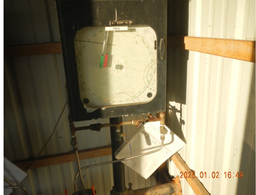
4. Gas meter inside meter shed at shared gathering location.
