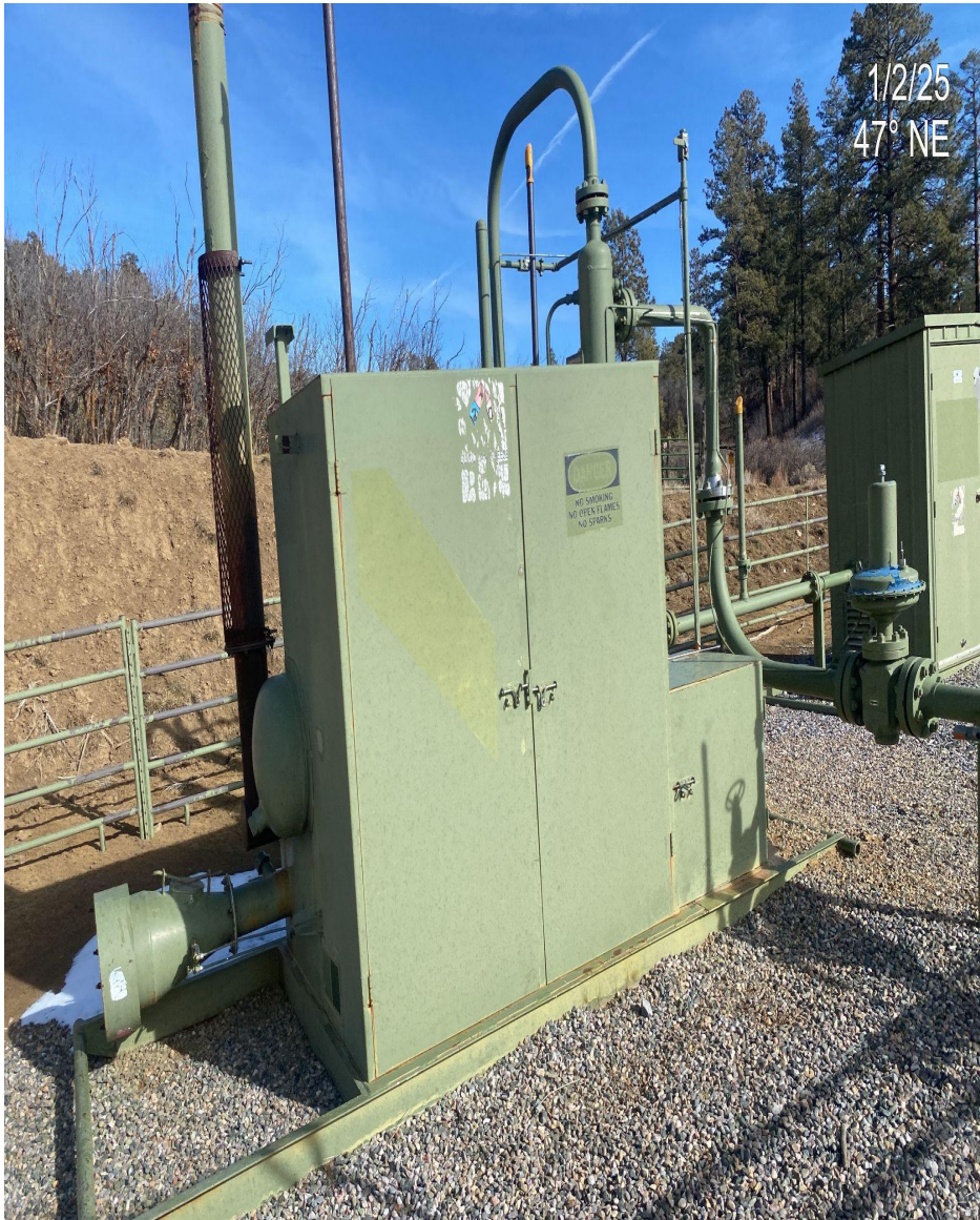
Photo 4. Signs/placards at separators have deteriorated and are no longer legible.
