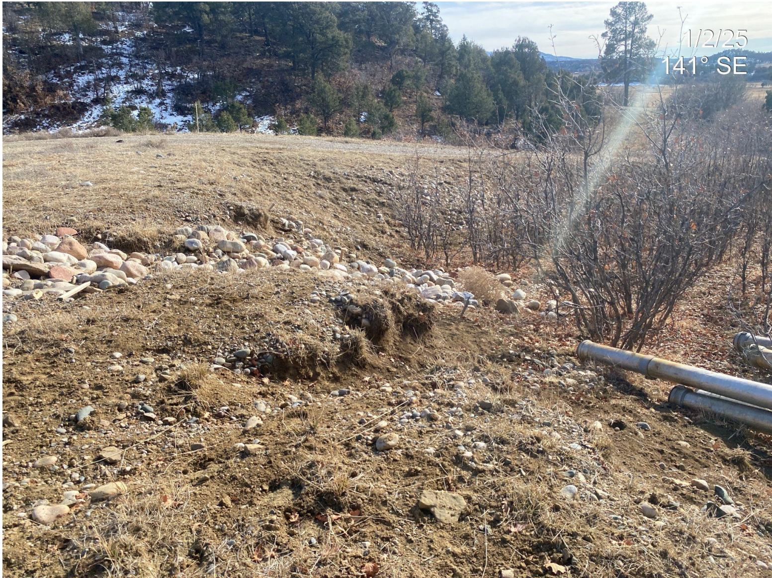
Photo 7. Erosion issues persist in the cut slope areas.
