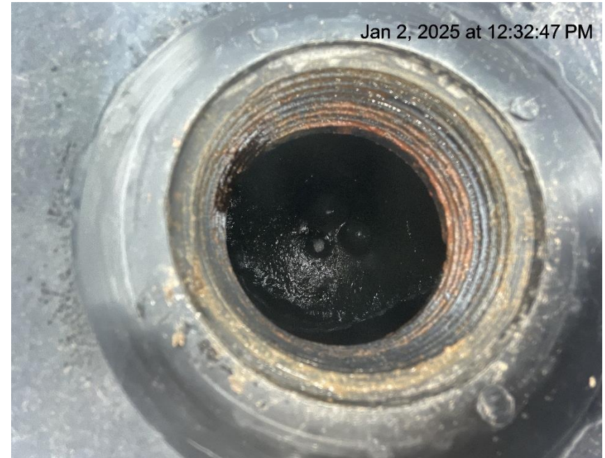
Photo # 6503 Failure to maintain chemical BMP – Chemical tank containment approximately 2/3 to 3/4 full of fluid/BMP insufficient to contain possible spill
