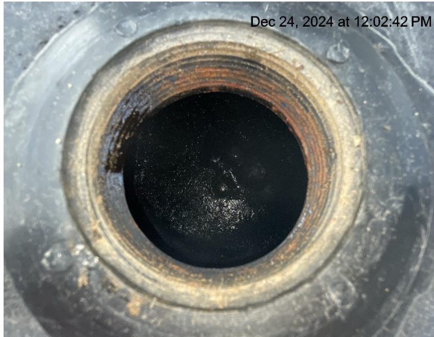
Photo # 5283 From inspection 708905317 conducted on 12/24/2024 Failure to maintain chemical BMP – Chemical tank containment approximately 2/3 to 3/4 full of fluid/BMP insufficient to contain possible spill
