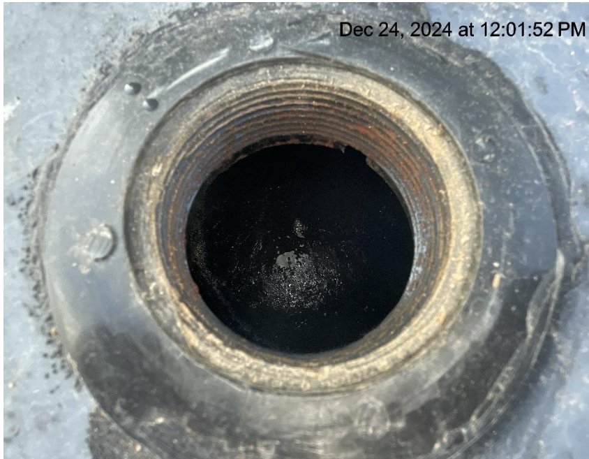
Photo # 5282 From inspection 708905317 conducted on 12/24/2024 Failure to maintain chemical BMP – Chemical tank containment approximately 2/3 to 3/4 full of fluid/BMP insufficient to contain possible spill
