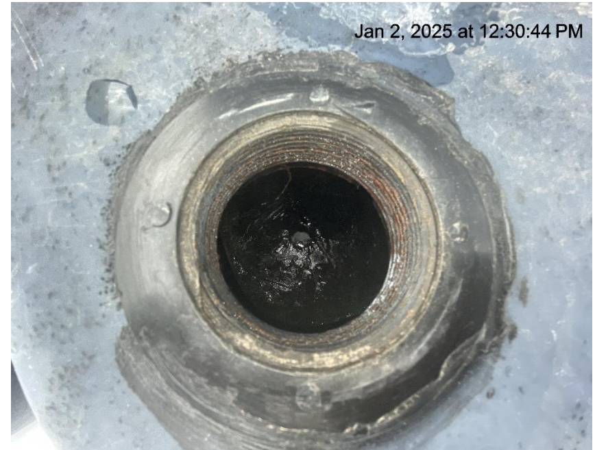
Photo # 6502 Failure to maintain chemical BMP – Chemical tank containment approximately 2/3 to 3/4 full of fluid/BMP insufficient to contain possible spill
