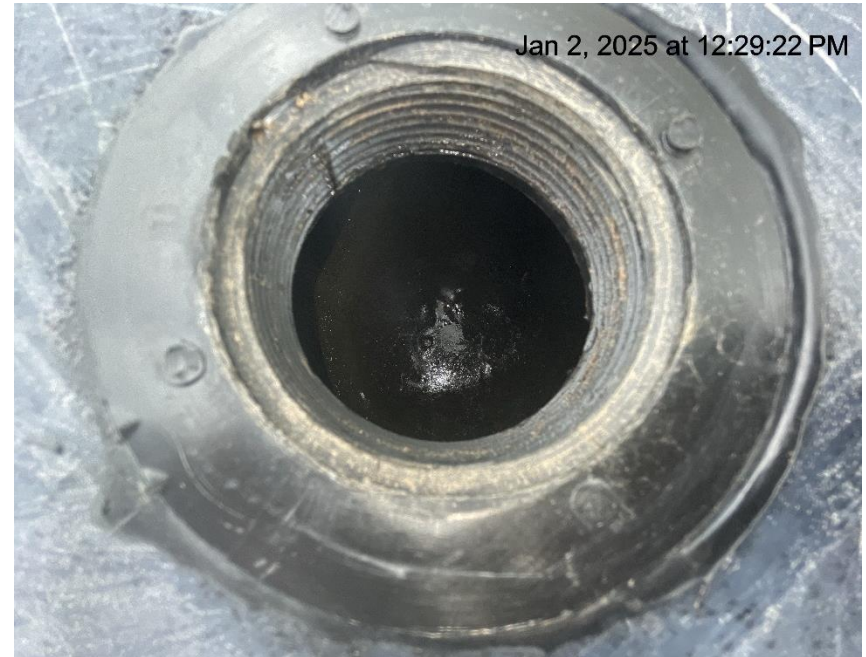
Photo # 6501 Failure to maintain chemical BMP – Chemical tank containment approximately 2/3 to 3/4 full of fluid/BMP insufficient to contain possible spill
