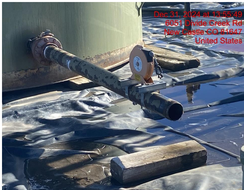
Open-Ended Line/Unused Equipment – Photo #05737
