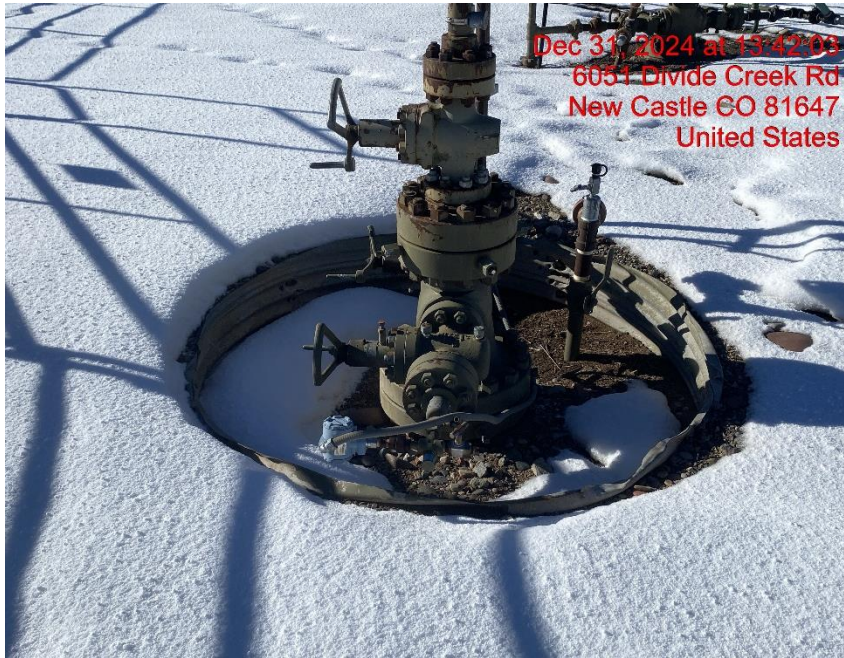
Open Wellhead Cellar/No Wildlife Egress – Photo #05716
