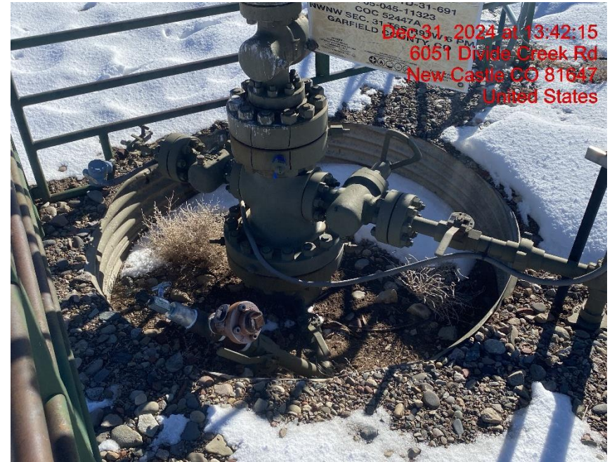
Open Wellhead Cellar/No Wildlife Egress – Photo #05717
