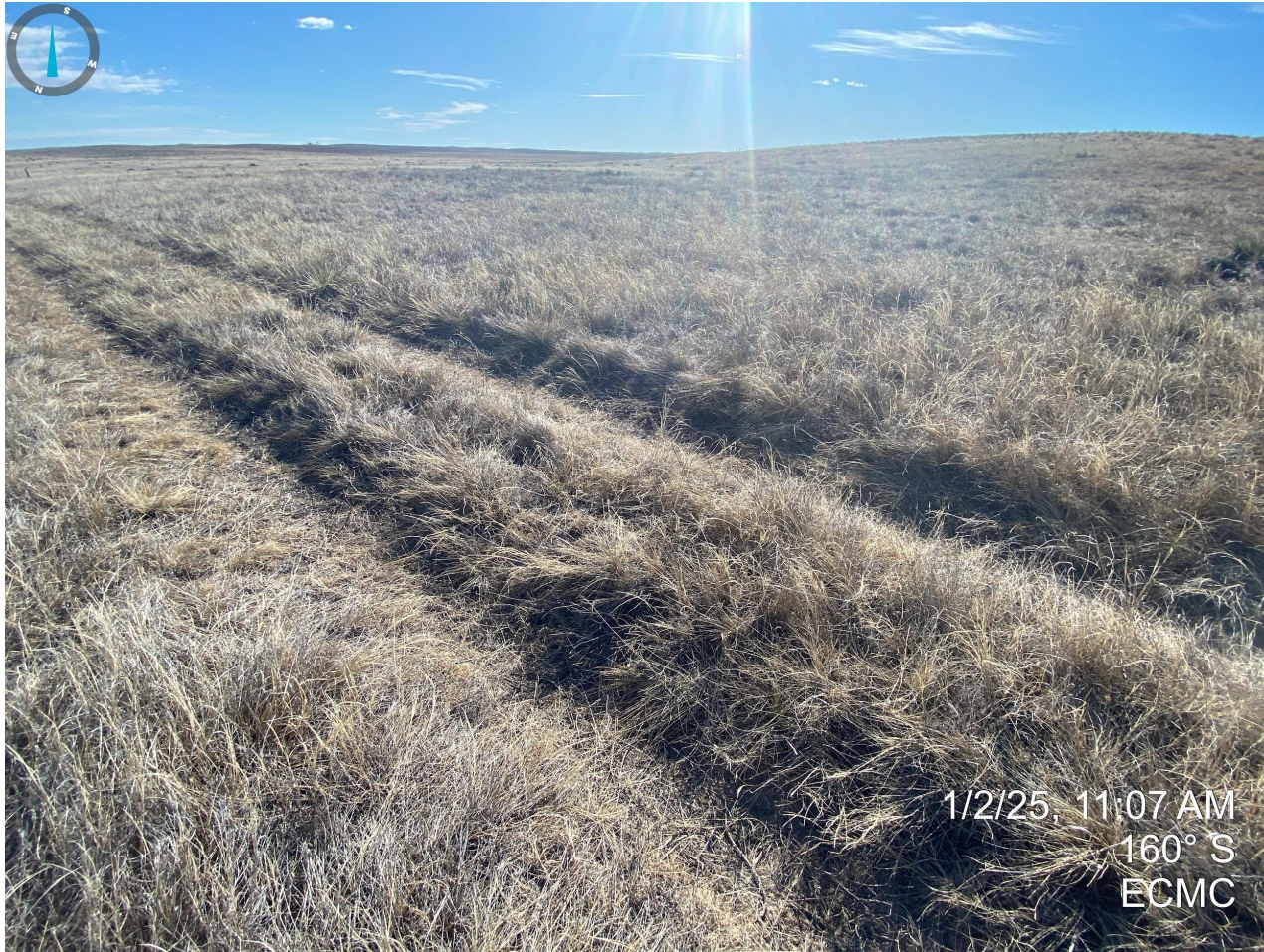
Photo 6. Access road Photo taken west of the location. Photo illustrates that portions of the access road do not appear to have been recontoured/graded to match the adjacent topography with ruts evident.
