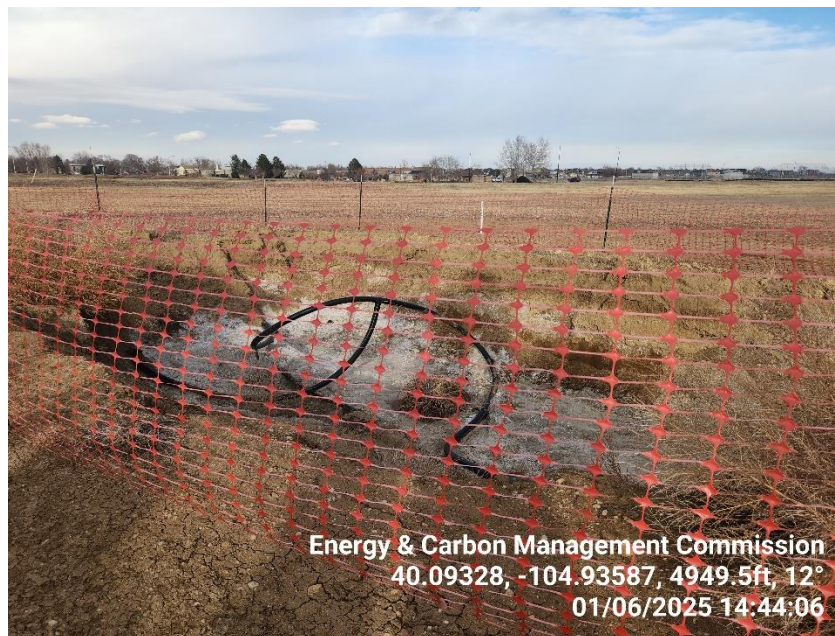
Photo 5 Unfinished flow line repairs in an open excavation.
