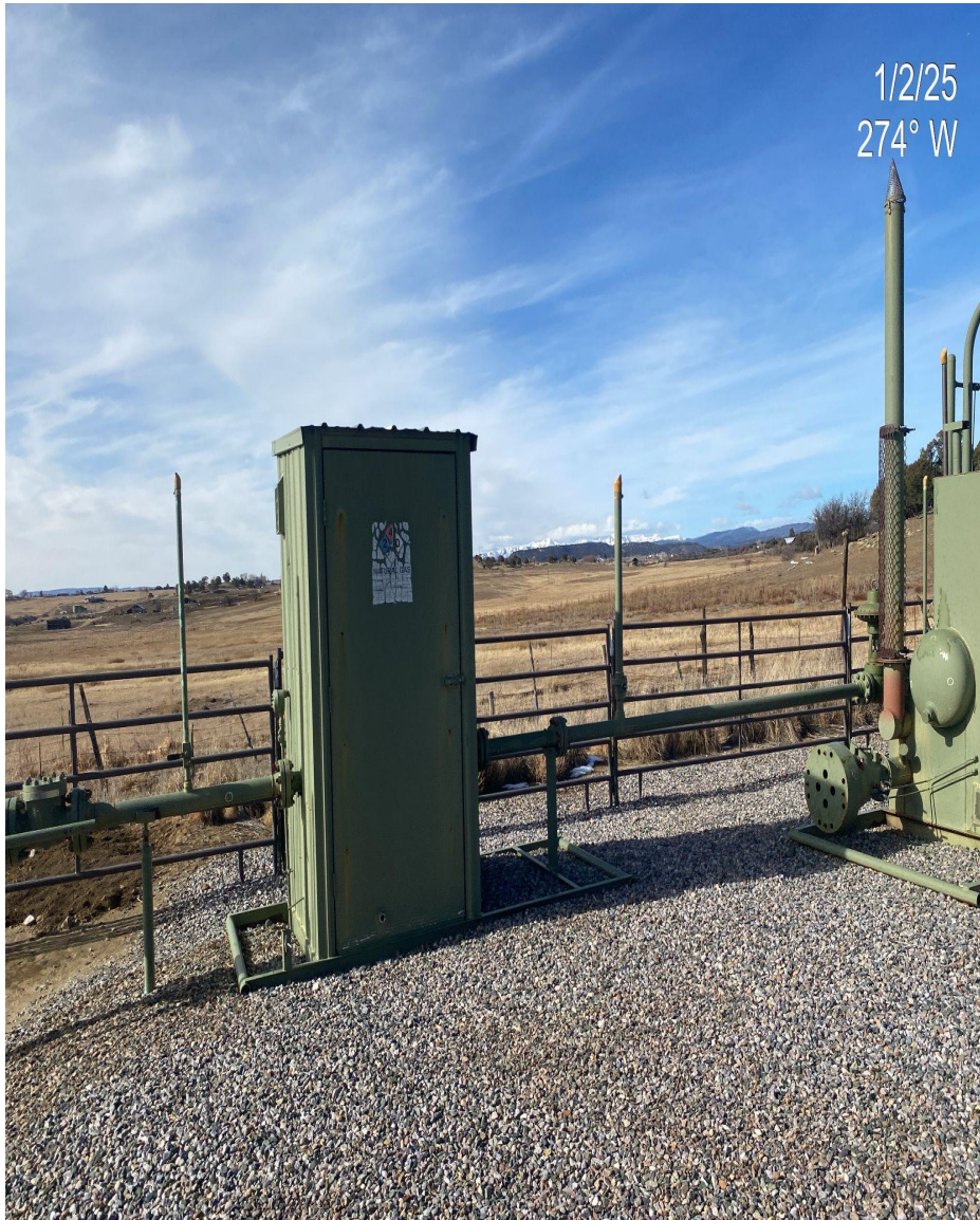
Photo 3. Signs/Placards at separator have deteriorated and are no longer legible.
