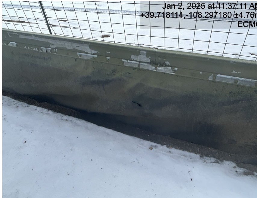
Hole in containment
